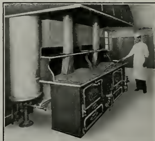
Crude Oil Burners Operating Kitchen Ranges in Government Barracks at Fort Winfield Scott
