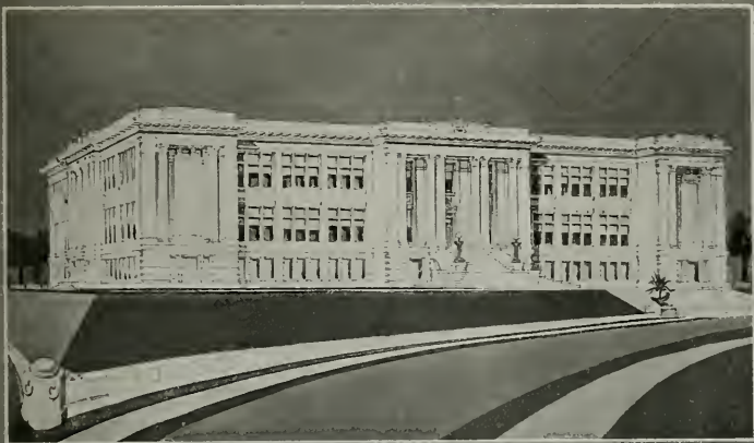
SANTA CRUZ HIGH SCHOOL, NOW UNDER CONSTRUCTION WILLIAM H. WEEKS, Architect
