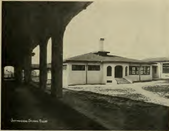
JEFFERSON SCHOOL BUILDING, OAKLAND, CALIFORNIA
