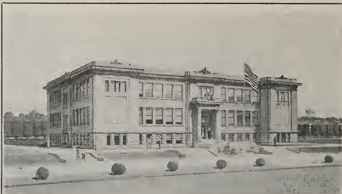
WILLOWS HIGH SCHOOL BUILDING, WILLOWS, CAL. W. H. WEEKS, Architect
