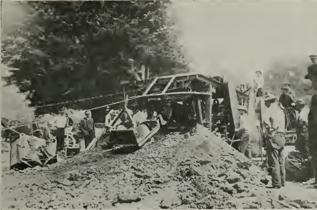
THE YOUNGER EXCAVATOR IN OPERATION
