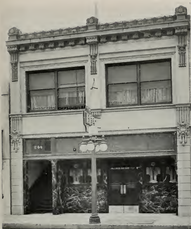
THOMAS BROWN BUILDING, MONTEREY, CALIFORNIA Wm. H. Weeks, Architect
