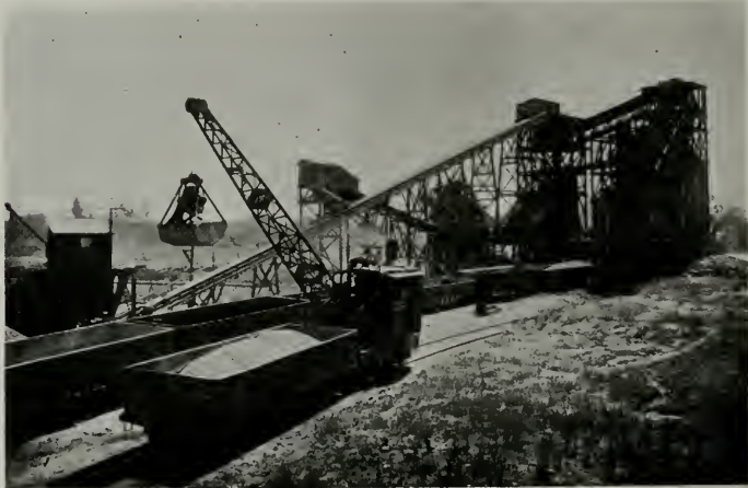
(Fig. D)—Port of plant of Niles Sand, Gravel & Rock Company, showing bunkers, loading facilities and locomotive crane in operation
