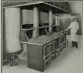
Crude Oil Burners Operating Kitchen Ranges in Government Barracks at Fort Winfield Scott
