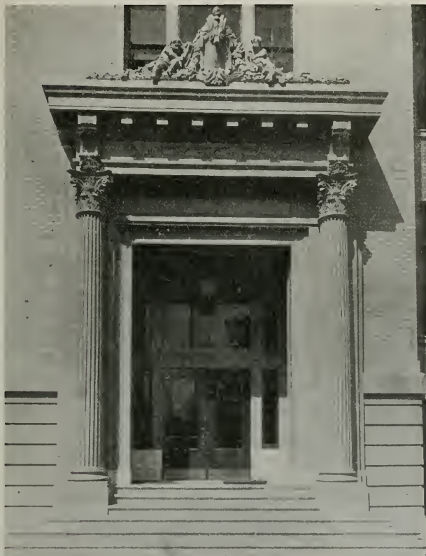
Detail of Entrance, Willows High School
