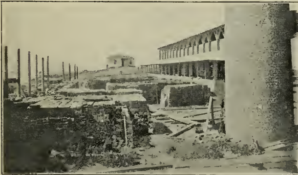
PAVING AND RED PRESSED BRICK AT VALLEJO BRICK & TILE CO.'S VALLEJO YARD
