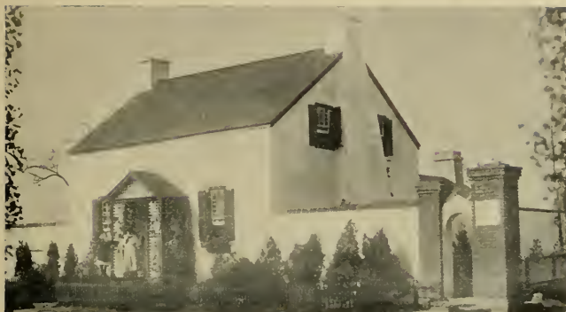
COTTAGE WITH 12-IN. CONCRETE WALLS BUILT FOR $2,450
