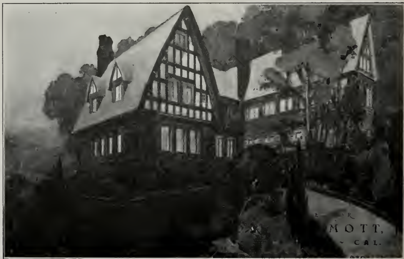
RESIDENCE, GEORGE M. MOTT, JR., CLAREMONT Warren C. Perry, Architect
