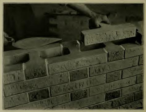
Fig. 13.—"An interesting version of an old well balanced Flemish band." Can be laid twice as fast as ordinary Flemish walls.
