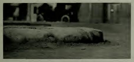
SPALLING OF GRANITE CURBING FROM TRAFFIC
