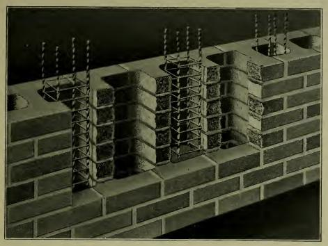
Fig. 7.—Thermos wall cut open to show the vertical air-spaces and columnor reinforcing.
