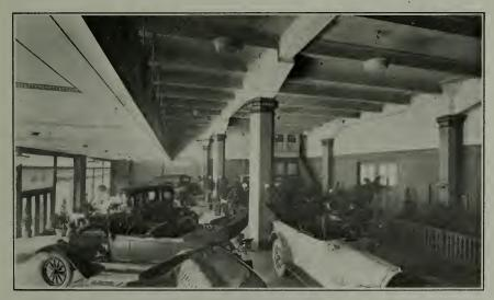
BUILDING FOR LOCOMOBILE COMPANY, SAN FRANCISCO Showing Heavy Concrete Beam and Girder Construction
