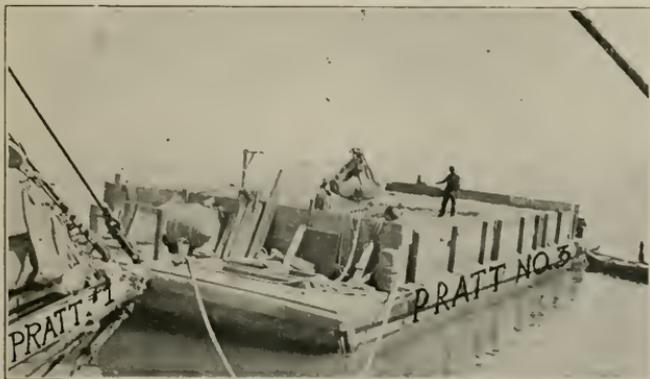
Unloading part of a 5,000 yard (equal to 200 car loads) order of washed gravel with clamshell bucket at Bolinas Bay for the J. G. White Engineering Corporation
