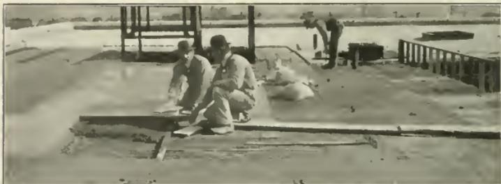
**Ferroidlave** ROOFS are erected without using forms
