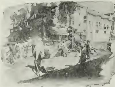
No. 6A Mixer with Gravity Distributing Chute on paving
