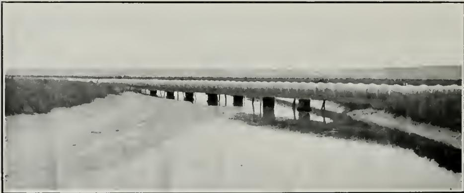
*Cut Shows Vitrified Clay Pipe Line Built Above Ground*
