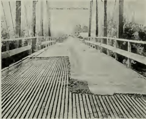
The Timber is Protected from the Rains and will Not Decay. It lessens the impact of the moving load on the structure.
