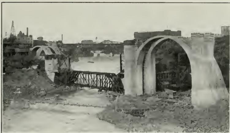
*Fig. 1 View Showing Spokane Arch With Steel Trusses in Place to Receive 281-Foot Timber Center*
