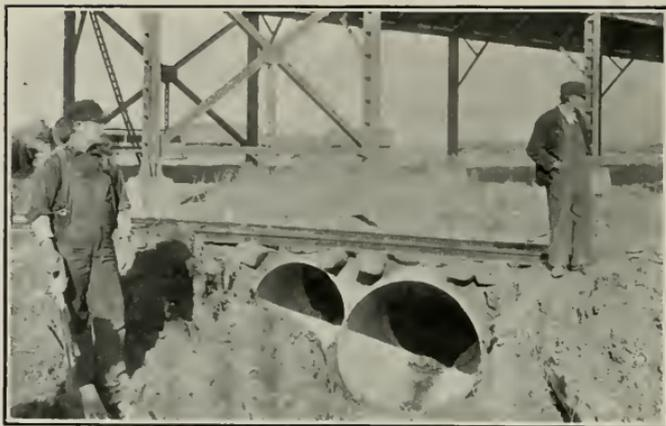
*Fig. 1. Showing Ingot Iron Culverts, one 36 inch and the other 46 inch
