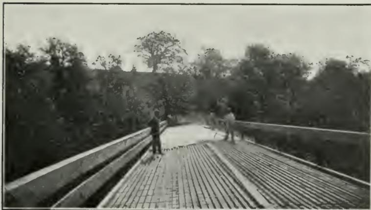
*Fig. 2, Showing Timbers Placed Lengthwise of the Bridge, and Concrete Wearing Surface on Deck Span*
