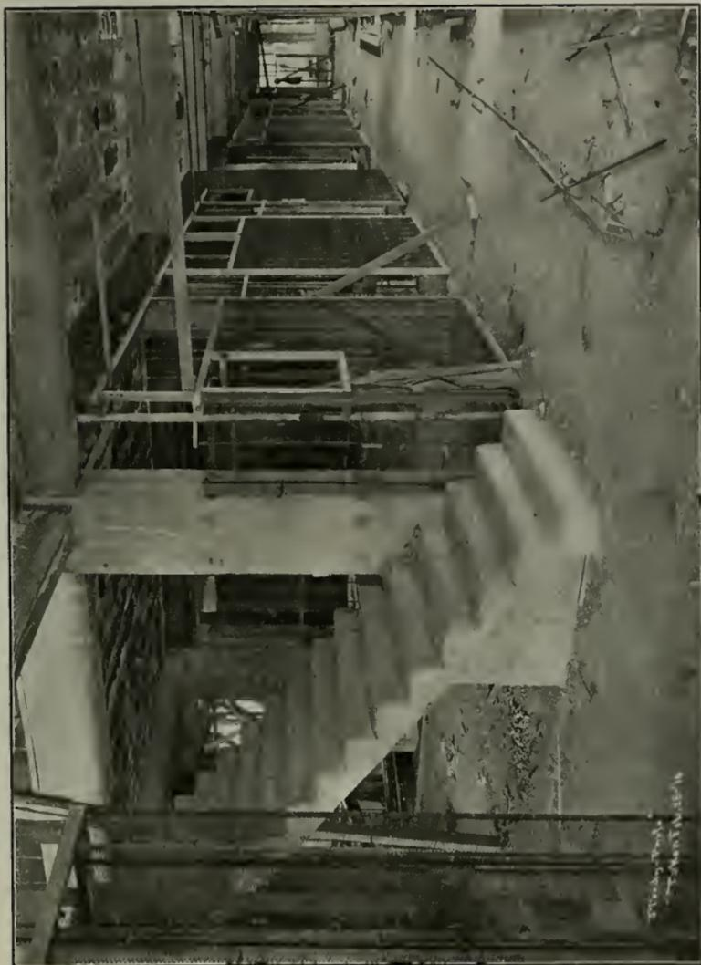
*Photo Showing Metal Partitions Before Plastering*
