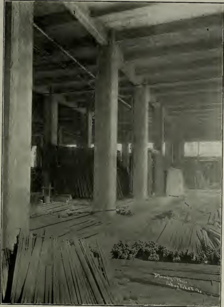
*Photo of First Floor After Removal of Forms, Showing Slab and Beam Systems of Construction.
