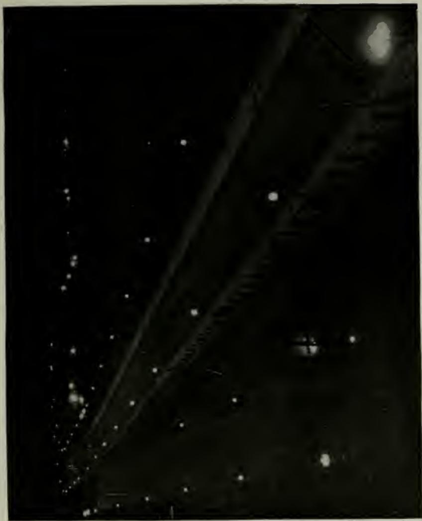
Fig. 2.—Night Scene on the Harrisburg Bridge. Note the Absence of Shadows Along the Entire Bridge. Compare the Effect of the Diffused Light with the Concentrated Glare and Surrounding Blackness as Indicated by the White Spots Which Are Arc Lamps in the Railroad Yards in the Background.
