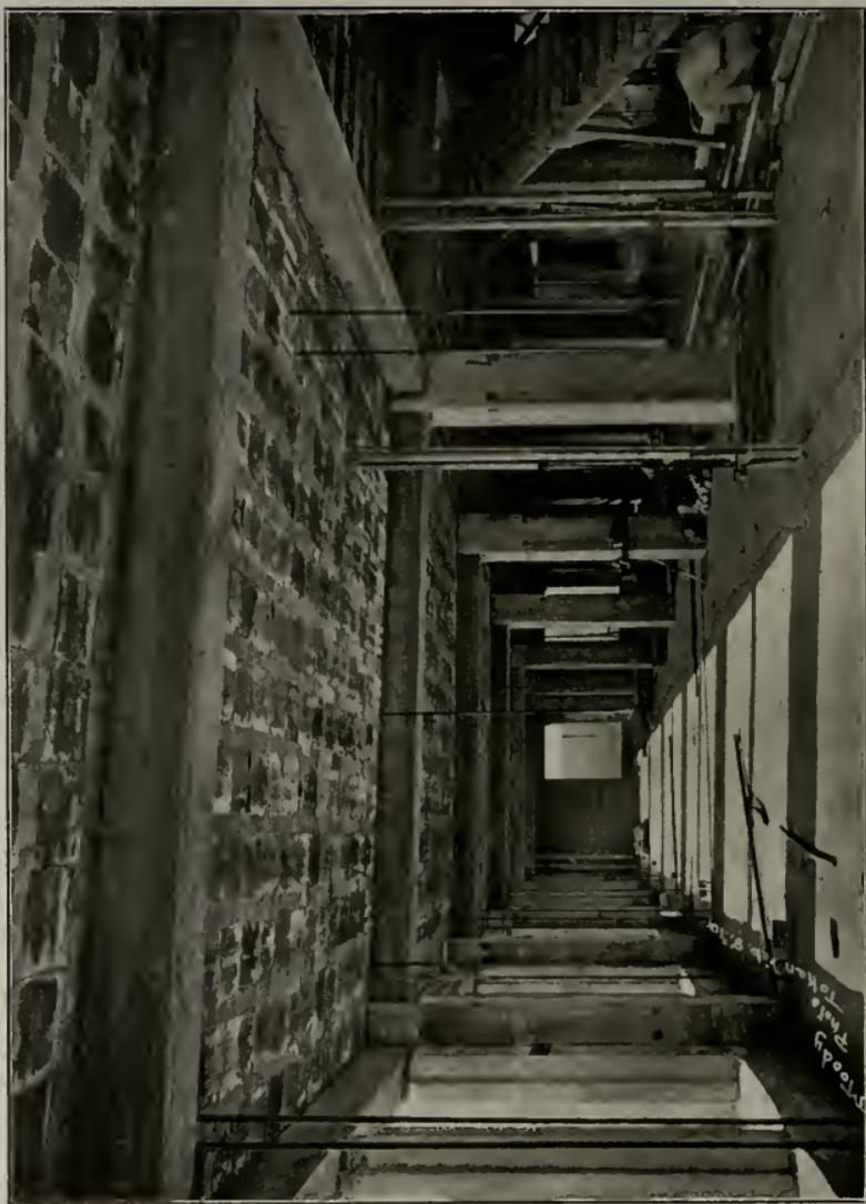
*Thomas Higgins Building—Showing Tile Construction After Forms Were Removed on Second Floor*
