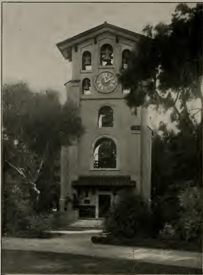
PICTURESQUE BELL TOWER AT MILLS COLLEGE, CAL., OF REINFORCED CONCRETE
