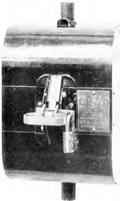
This switch is used in connection with all motors up to 5 H. P.
