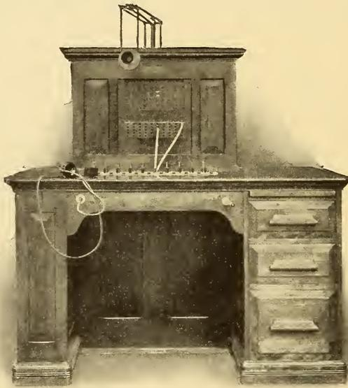
FIG. 316.—PRIVATE-BRANCH EXCHANGE SWITCH-BOARD.
