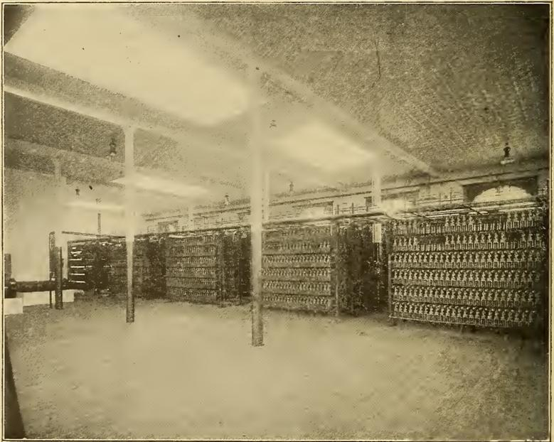
FIG. 520.—SWITCH ROOM IN GRAND RAPIDS AUTOMATIC EXCHANGE.
