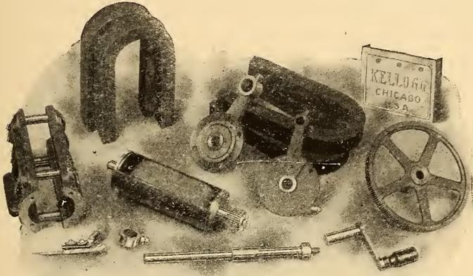
FIG. 95.—PARTS OF KELLOGG GENERATOR.
