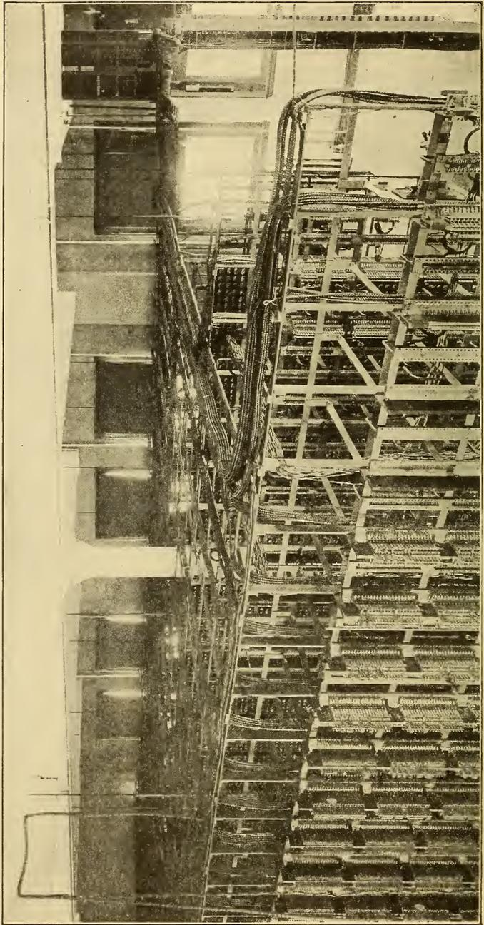
FIG. 481.—RACK ON TOP OF FRAMES—KEYSTONE TELEPHONE COMPANY.
