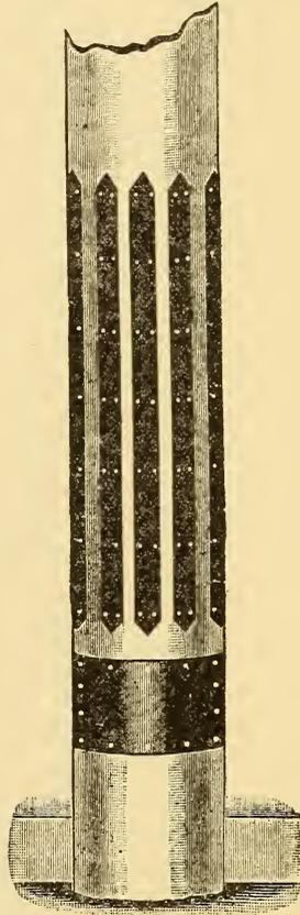
FIG. 536.—POLE STRIPS AND BUTT PLATES.
