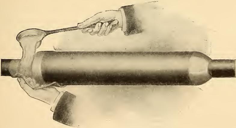
FIG. 604.—CABLE SPLICING.
