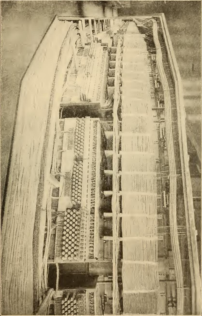
and supervisory relays, and at the bottom of the view is the mass of intermediate-to-answering cables, these cables lying in a running box on the floor, a portion of which is removed in this view for the purpose of giving a better view of the cables themselves.
