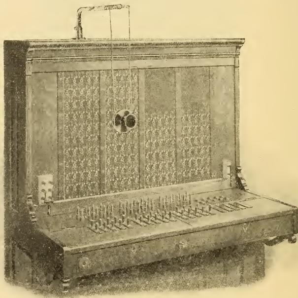
FIG. 193.—TWO-POSITION SWITCH-BOARD.
