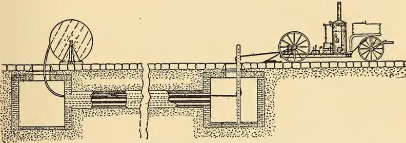
FIG. 620.—DRAWING IN BY STEAM POWER.
