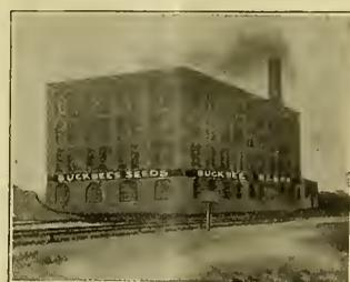
three railroads passing along two sides of the building. The building is so arranged that the seeds are taken in on the first floor and then carried by elevators to the portions of the building where they belong.
