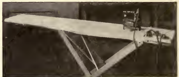
The ironing board in use. It is not necessary to conceal the wiring for conveniences not classed with furniture
