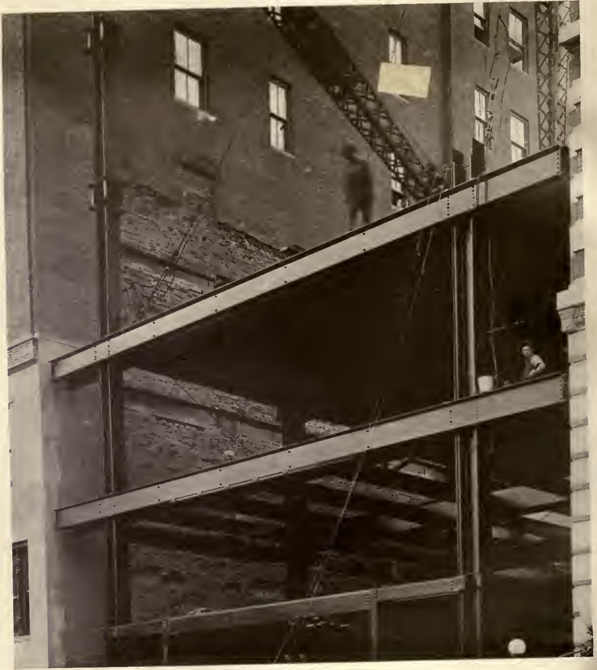
A loft building, 66-70 West 40th Street, New York City, with side walls carried on cantilever ends of floor girders Necarsulmer & Lehlbach, Architects Gunvald Aus Company, Engineers
