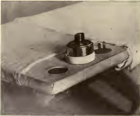
The ironing board has a socket to receive plug from nearby outlet; an outlet for the attachment of the iron and a switch between to insure safety
