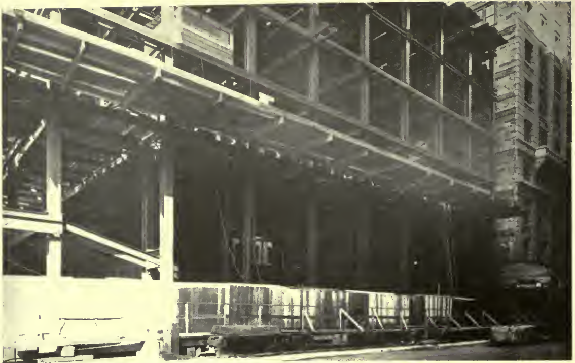
PROGRESS VIEW. SLOPING STEEL WORK FOR BALCONY CAN BE SEEN AT THE LEFT
