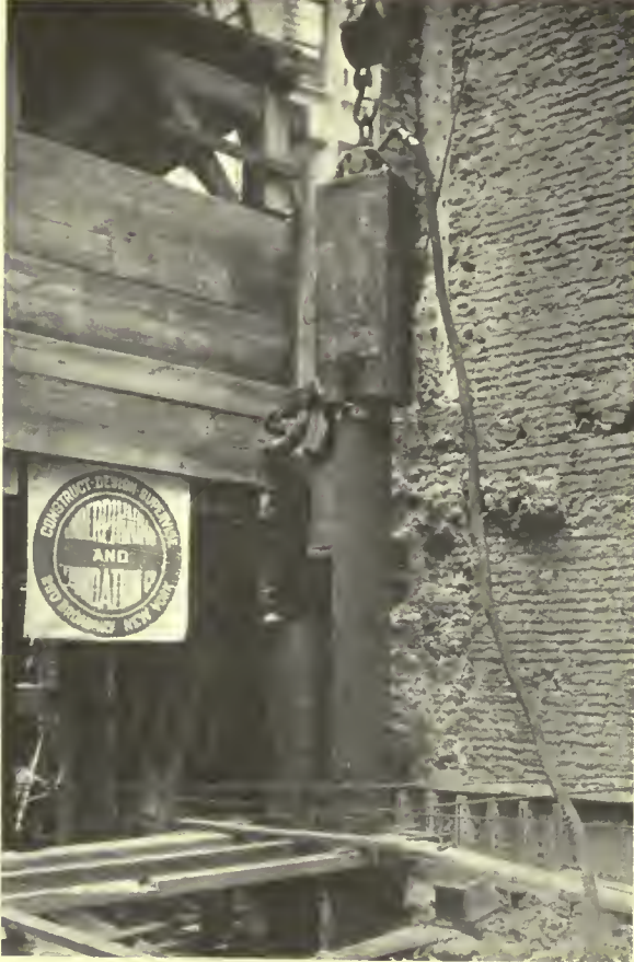
DRIVING TUBULAR PILES CLOSE TO AN EXISTING WALL BY STEAM HAMMER
