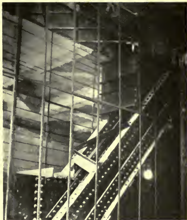
METHOD OF FIREPROOFING STEEL TRUSSES
