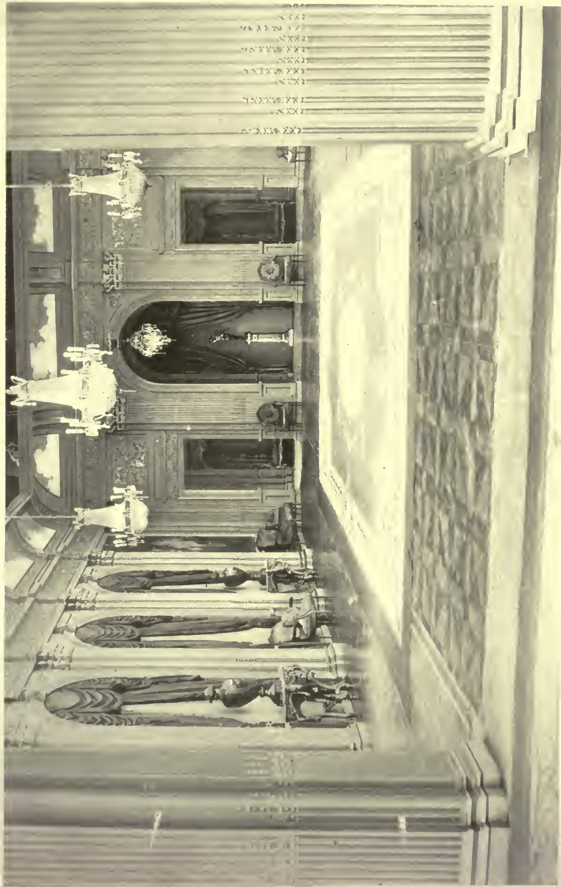
A MOTION PICTURE SET, DESIGNED AND EXECUTED UNDER THE DIRECTION OF ROBERT HAAS, ARCHITECT A salon of the Elysee Palace, Paris, reproduced on the studio floor. This room occupies a space 80 by 120 feet. The walls are of wood ornamented with plaster. Note the presence of the ceiling cove and absence of a ceiling proper.
