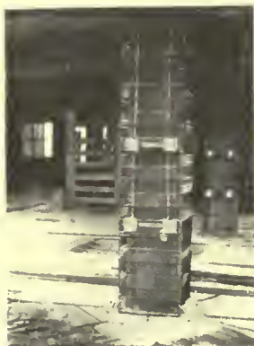
Outer Wrapping of Metal Lath
