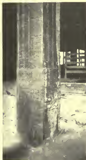
Inner Wrapping of Metal Lath
