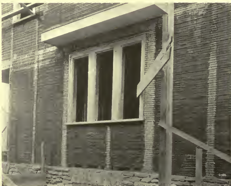
FIG. 4. EXTERIOR VIEW SHOWING PAPER AND REINFORCEMENT IN PLACE. Concrete studs and beams have just been cast.
