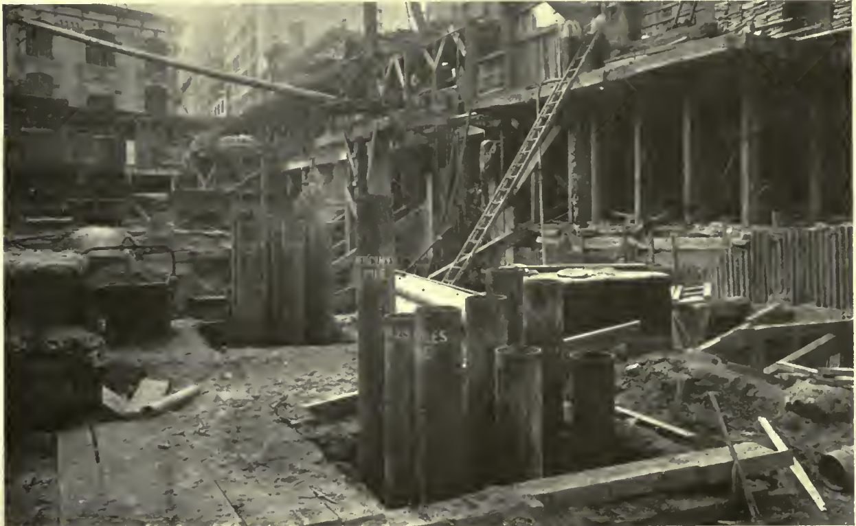
A FOUNDATION IN WHICH HERCULES TUBULAR PILES, DRIVEN TO ROCK, WERE USED That part of the steel tube which projects above the specified level is cut off by the use of the oxy-acetylene burner
