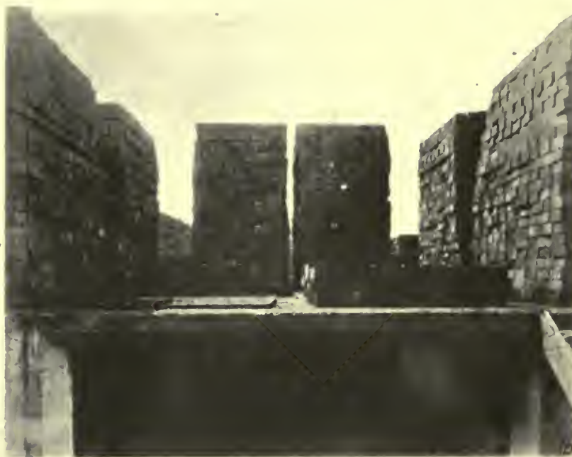
CLOSE-UP VIEW OF SLAB UNDER FINAL LOAD
