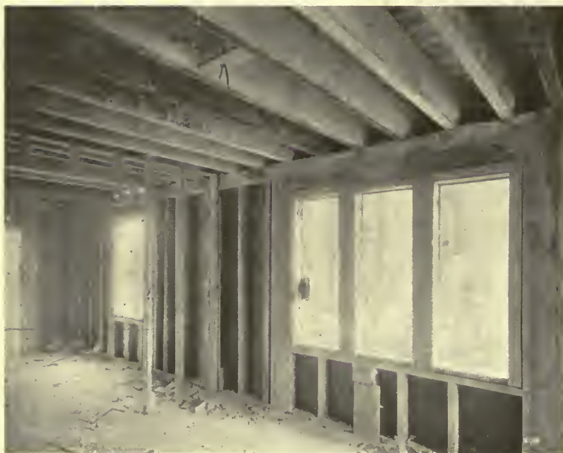
FIG. 3. INSIDE VIEW OF WALL, SHOWING CONCRETE STUDS, ALSO SPECIAL LINTEL OVER TRIPLE WINDOW
