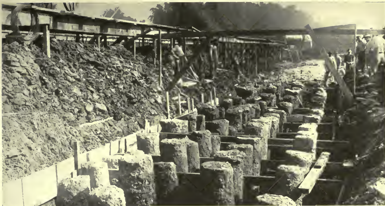
GROUP OF PEDESTAL PILES FOR THE WILLYS-OVERLAND COMPANY'S PLANT AT TOLEDO, OHIO Earth around tops of piles excavated and forms being placed for concrete cap
