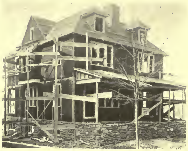
FIG. 6. OUTSIDE REINFORCEMENT ENTIRELY IN PLACE
