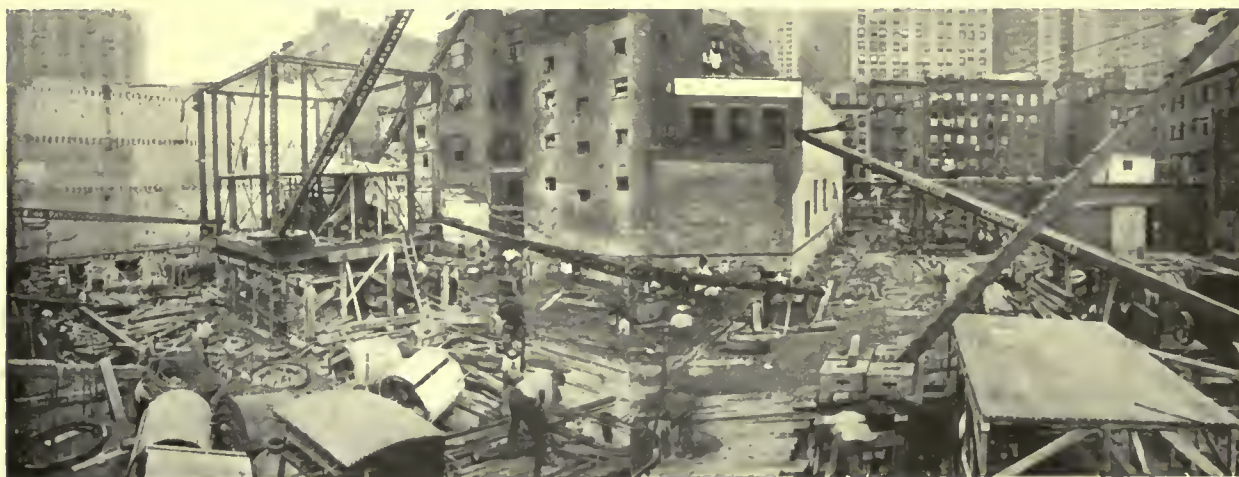
COMMENCEMENT OF FOUNDATION WORK ON THE BARRETT BUILDING, NEW YORK CITY Note cutting edges with vertical reinforcement (at left) in place for circular caisson construction
