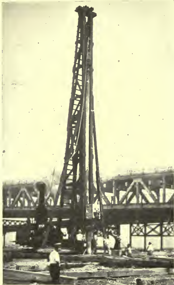
APPARATUS USED IN DRIVING PEDESTAL PILES
