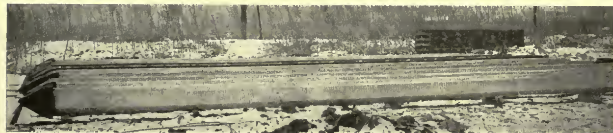
GROUP OF GIANT PRECAST CONCRETE PILES IN PROCESS OF SEASONING PRIOR TO DRIVING
