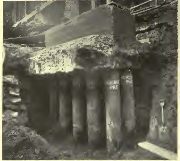
GROUP OF TUBULAR PILES PARTIALLY EXPOSED
