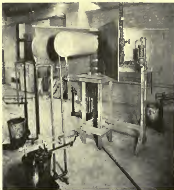
FIG. 2. PHOTOGRAPH SHOWING THE PRINCIPAL OPERATIVE FEATURES OF THE STEAM DRUM PLANT
