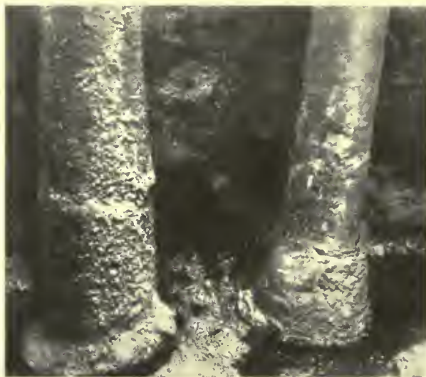
TWO PEDESTAL PILES, EXCAVATED FOR INSPECTION
