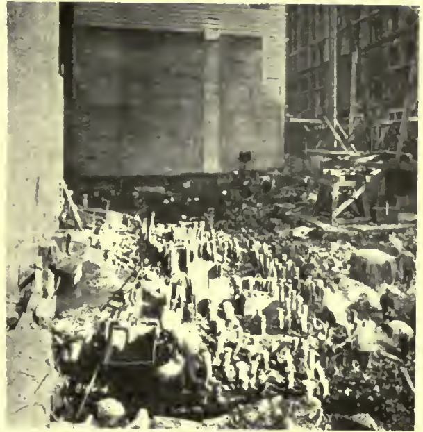
CHURCH EDIFICE ENTIRELY REMOVED Site was excavated to rock and all old piling removed.
