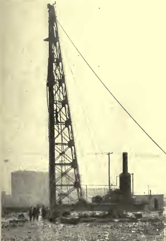
ALL METAL PILE DRIVER AND 60-H.P. ENGINE.
