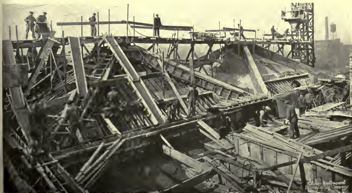
UNUSUAL ROOF CONSTRUCTION—NOTE REINFORCED CONCRETE HIP GIRDERS N. MAX DUNNING, ARCHITECT. LIEBERMAN, KLEIN & HEIN, ENGINEERS
