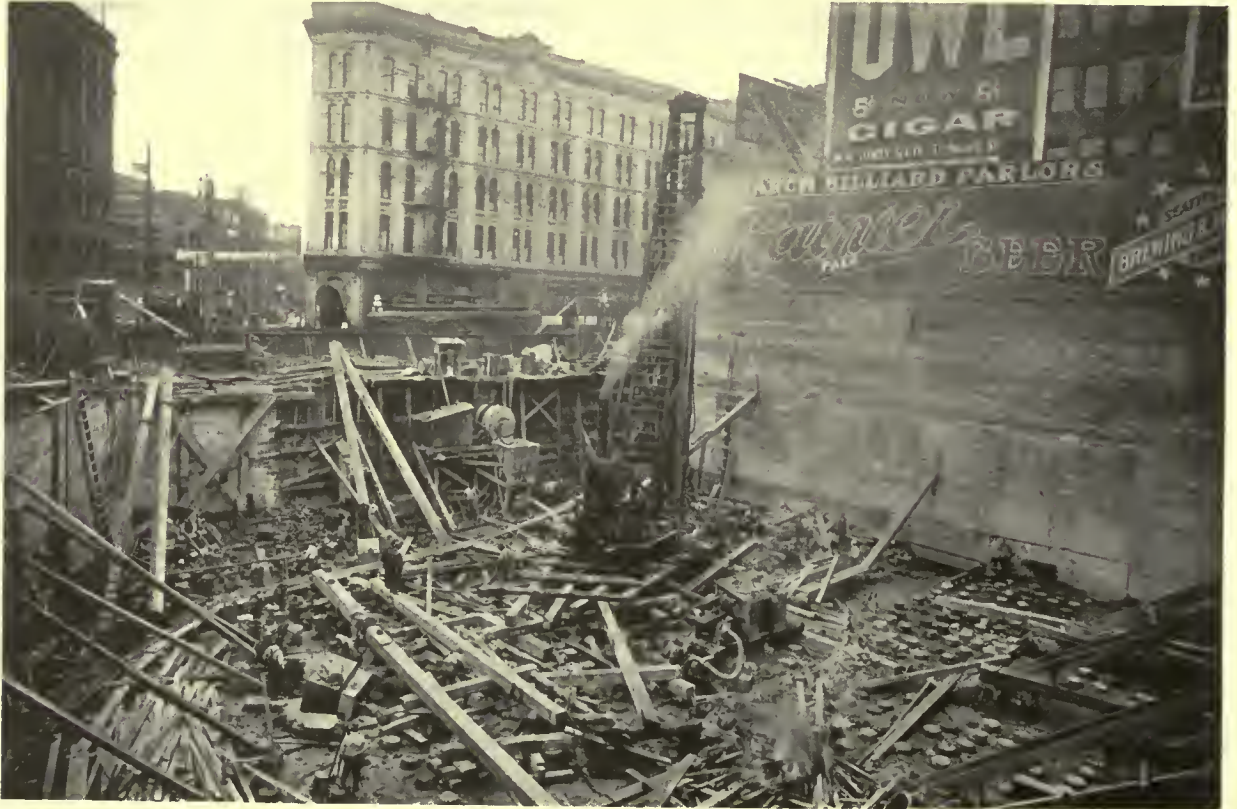
PILE DRIVING IN PROGRESS FOR THE L. C. SMITH BUILDING, SEATTLE, WASH.
