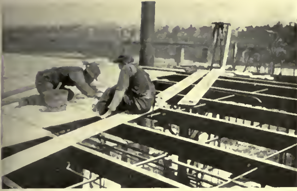
ROOF CONSTRUCTION—STEEL CHANNELS AND POROUS SLABS
