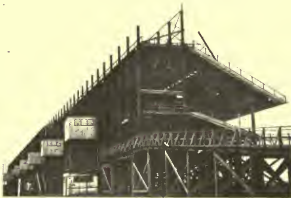
THE GRANDSTAND, WHICH PROVIDED SEATING ACCOMMODATIONS FOR 35,000 PERSONS, IN COURSE OF DEMOLITION
