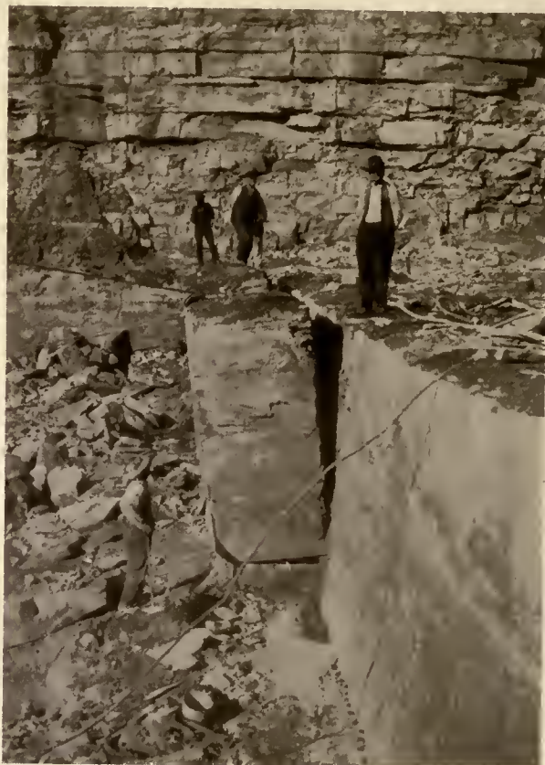
TURNING OVER "CUT" IN QUARRY AFTER BEING CUT OR CHANNELLED BY CHOPPING OR CHANNELING MACHINE
