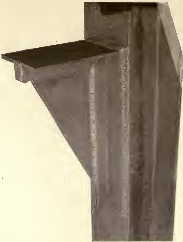
BRACKET SUPPORT FOR 5-TON CRANE RAIL, JOINED TO COLUMN BY ELECTRIC ARC WELDING
