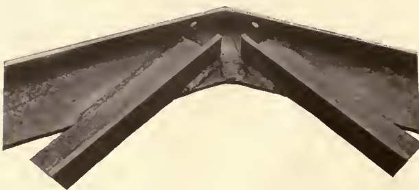
WELDED CONNECTION AT PEAK OF TRUSS
