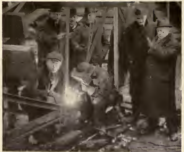
MAKING AN ELECTRIC ARC WELD
