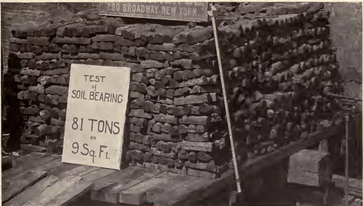
TESTING THE SOIL
