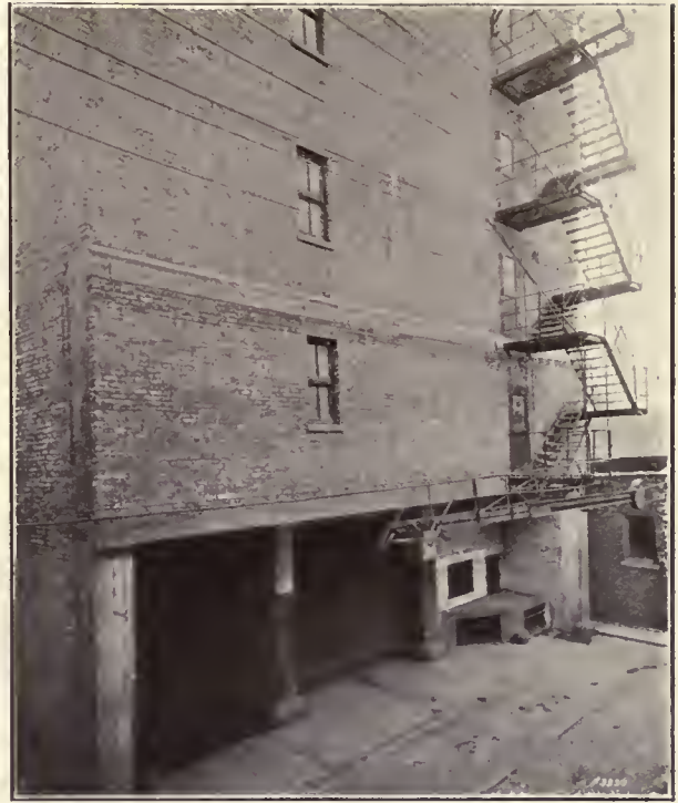
REAR ELEVATION SHOWING LOCATION OF RE-INFORCED CONCRETE TRUSS IN SECOND STORY
