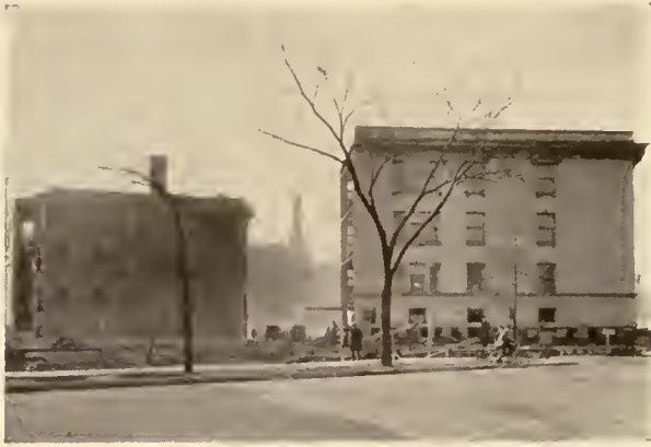
TURNING OF SECTION 2 ALMOST COMPLETED AND READY TO BE MOVED BACK INTO FINAL POSITION. SECTION 1 AT LEFT AND UNDERPINNED WITH BRICK ON NEW FOUNDATIONS. SECTION 2 STILL IN IRVING AVENUE, JACKSON BOULEVARD IN FOREGROUND.
