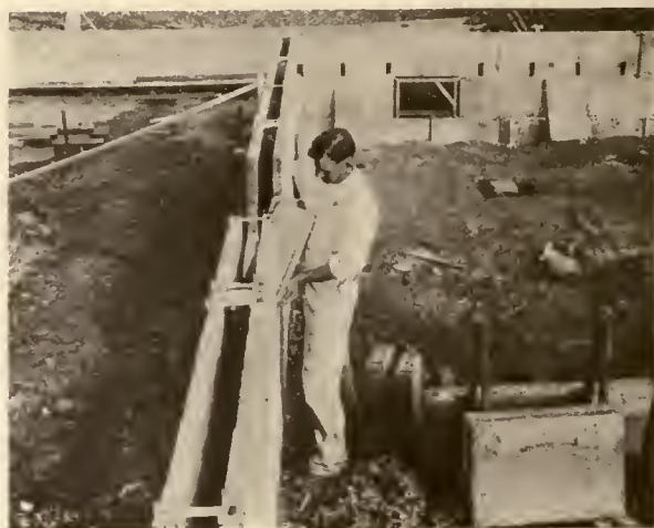
CONSTRUCTING A DOUBLE WALL WITH CONCRETE BLOCKS. IN THIS CASE THE AIR SPACE IS CONTINUOUS AND FURRING THE INTERIOR IS UNNECESSARY
