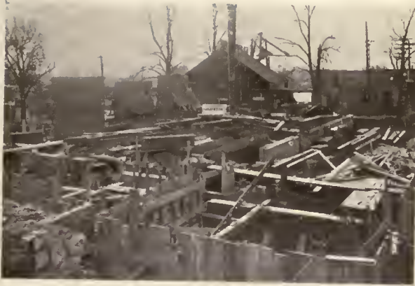
NO. 1. FOUNDATION WORK IN PROGRESS. SOME OF C. I. COL. BASES SET; PART OF STEEL ON JOB AND READY FOR ERECTION. BUILDING OF BRICK WALLS COMMENCED
