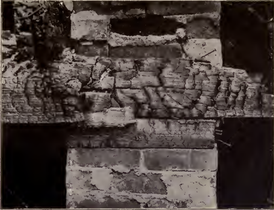
RESULT OF POOR CHIMNEY CONSTRUCTION. FLOOR ATTACHED TO CHIMNEY HAVING ONLY 4-INCH WALLS AND NO LINING. FIRE DESTROYED BUILDING
