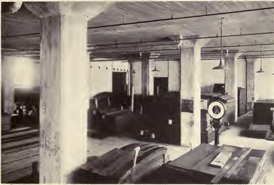
THE OAKES COMPANY BUILDING, INDIANAPOLIS VONNEGUT, BOHN & MUELLER, ARCHITECTS. INTERIOR VIEW SHOWING THE TEMPORARY DRAINS FROM THE ROOF.
