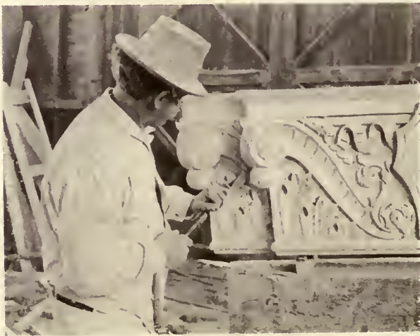
CARVING PILASTER CAPITOL. CARVER IS USING AIR-HAMMER
