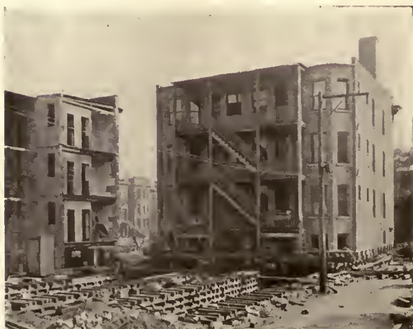
REAR OF SECTION 1 LOOKING EAST. THE BUILDING IS MOVED INTO IRVING AVENUE AND READY TO BE TURNED 180 DEG. ON ITS CENTER. TO THE LEFT IS REAR OF SECTION 2. NOTE THE SILLS, ROLLERS AND CRIBBING.
