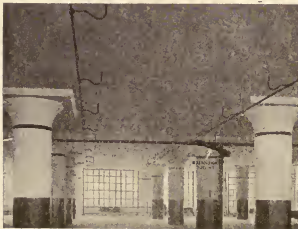
GENERAL VIEW OF SPRINKLER LINES. INSULATING ARMS AND EXPANSION JOINT CAN BE SEEN
