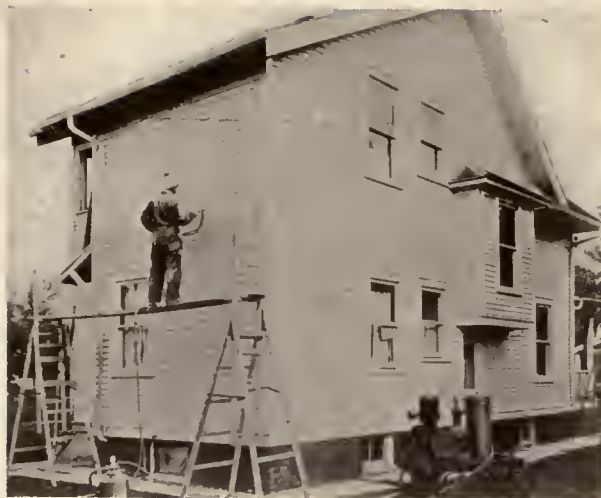
SPRAYING METHOD APPLIED TO SPRING HOUSE PAINTING
