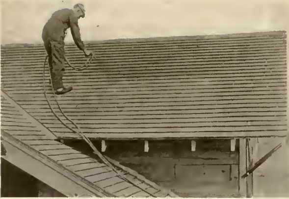
SPRAY PAINTING A SHINGLE ROOF Such surfaces often prove difficult for brush work
