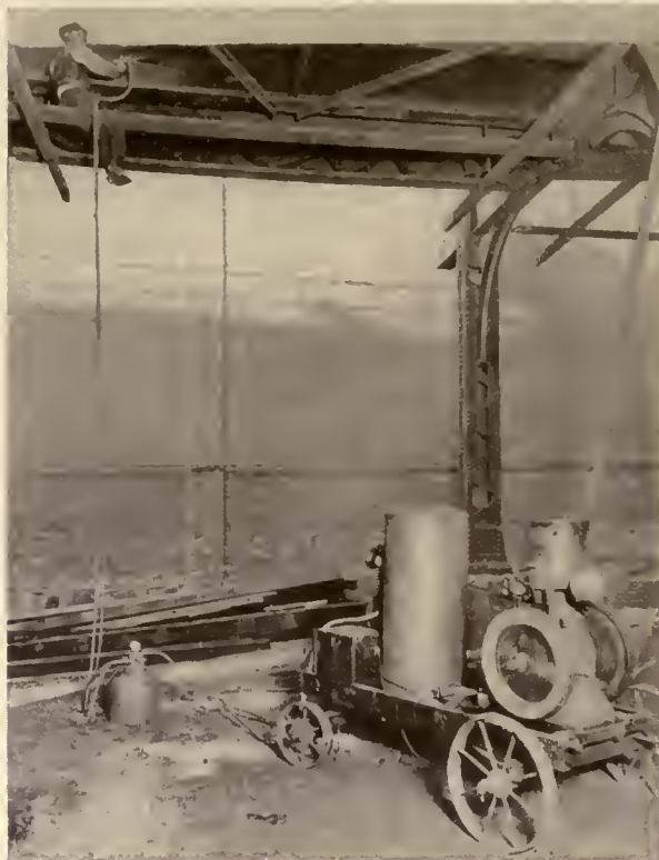
APPLYING PAINT TO THE STEELWORK OF AN ELEVATED RAILWAY STRUCTURE BY SPRAYING
