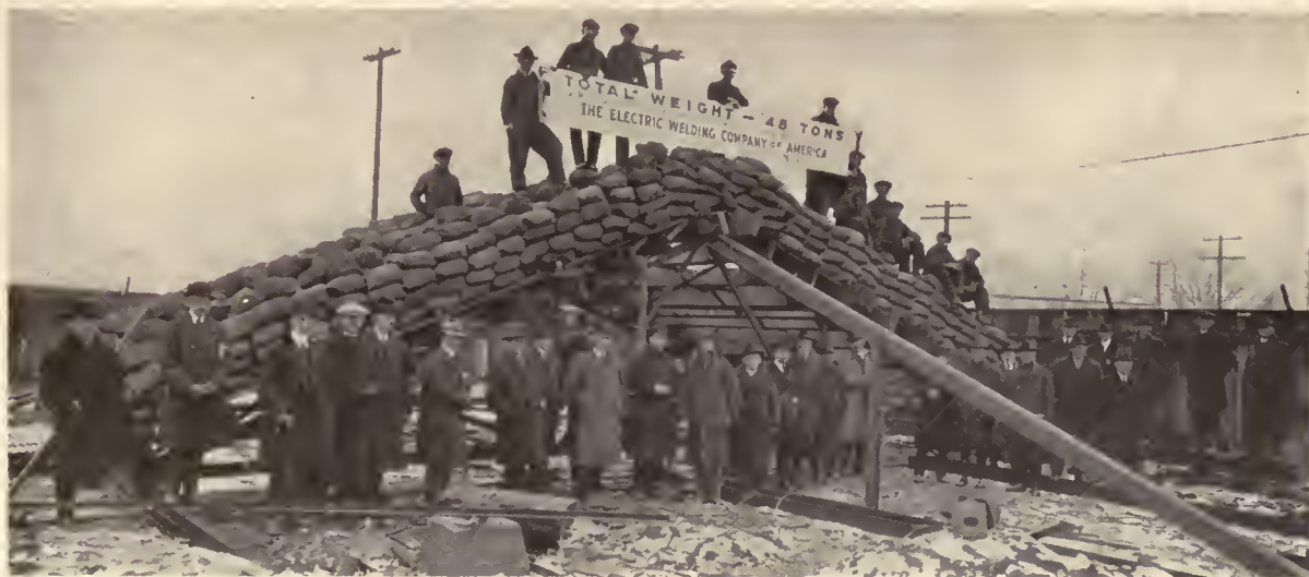
TWO ELECTRICALLY ARC WELDED TRUSSES SUPPORTING A 50 PER CENT OVERLOAD
