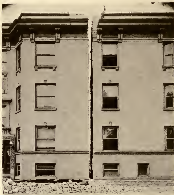
CUTTING THE BUILDING INTO TWO SECTIONS, SECTION 1 AT LEFT AND SECTION 2 AT RIGHT. SECTION 1 "LOADED" ON THE FALSEWORK READY TO BE RAISED PREPARATORY TO MOVING.
