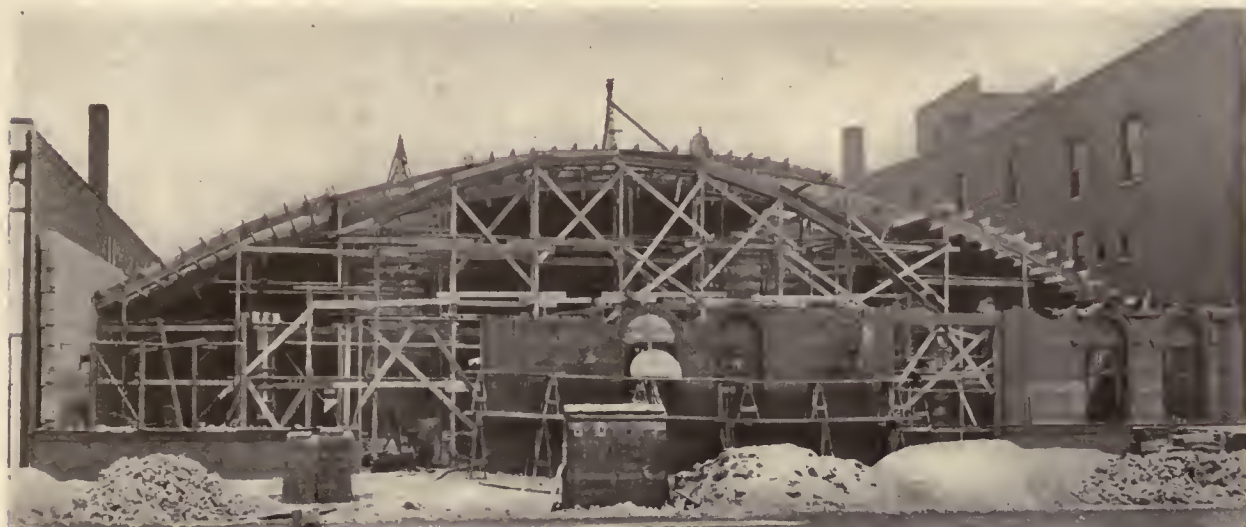
COTTAGE GROVE AVENUE END OF GARAGE DURING CONSTRUCTION. NOTE FALSEWORK SUPPORTING FORMS FOR CONCRETE ROOF ARCHES
