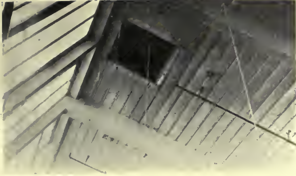
Fig. 20. Roof rotted for 10 or 15 feet from a ventilator, owing to the escape of heat, reducing the temperature and causing moisture to precipitate on the roof planks.
