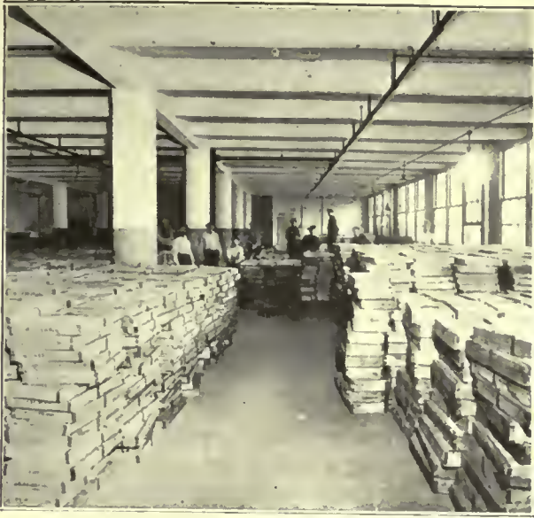
Interior view of second story showing heavy overload of tin. The work of removal has just been commenced.
