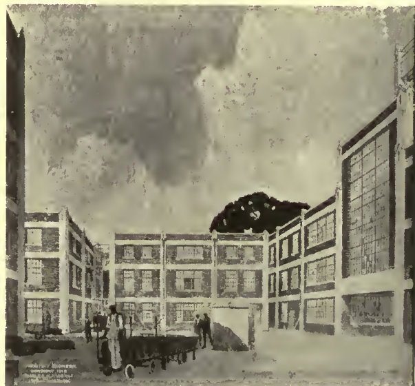
Perspective sketch of Building 7, showing exterior stairs and communication platforms connecting to Building 6 at the left. Building 10A, 10B at right, hose and hydrant house and motor truck in foreground.
