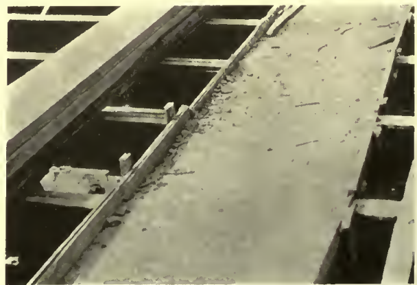
A reinforced concrete T-beam girder the forms of which are filled, the concrete enclosing the ends of the metal floor joists.
