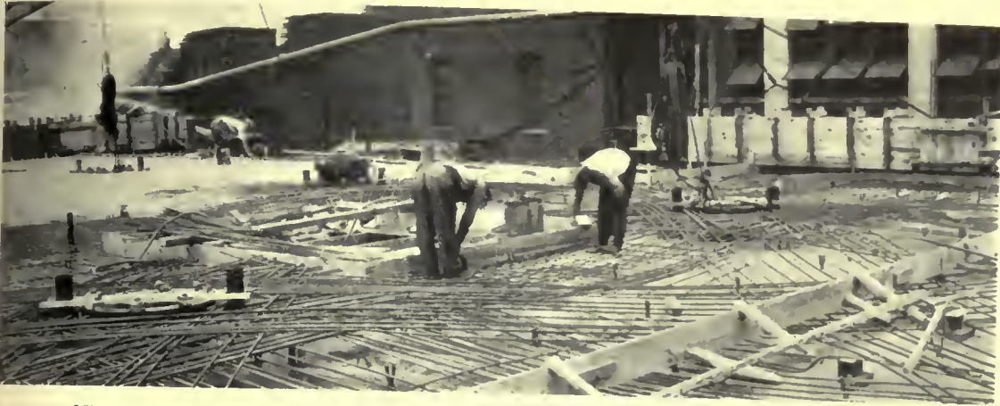
View of a partially poured concrete floor, showing the four-way reinforcing rods in place
