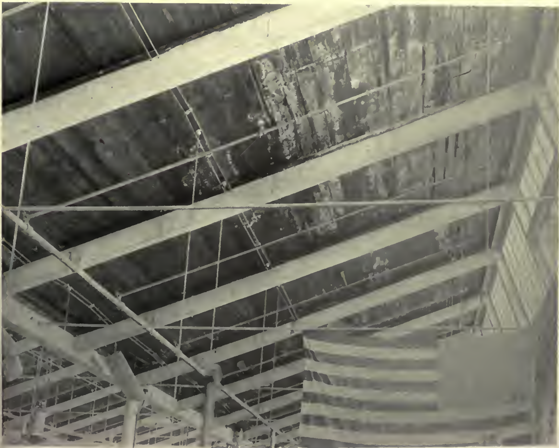
Fig. 15. Roof planks of a New Bedford weave-shed from which the sheathing has been removed. The planks were destroyed in nine years.
