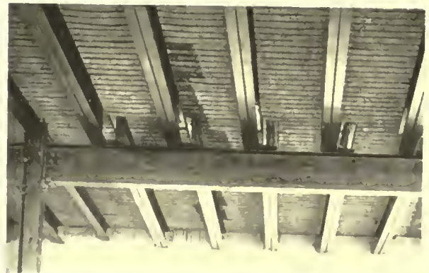
A floor with metal joists, structural steel girders and columns. Concrete floor slab in place. View from below.
