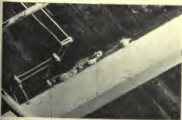
Fig. 6. Fomes Officianalis plants growing on the side of a beam under a weave-shed roof from which the sheathing has been removed for some time.
