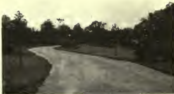
Photo 16.—Sharp entrance drive curves should be safeguarded by ample width of road-bed.
