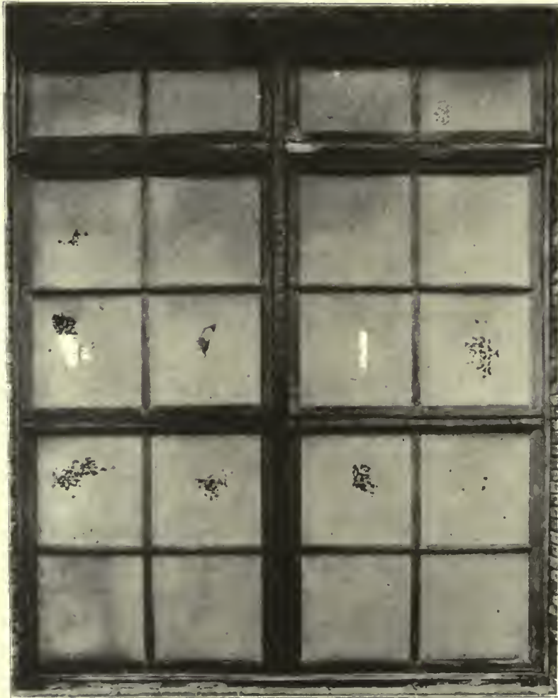
New type of fire window and transom having only a 2-in. mullion which tested out satisfactorily.
