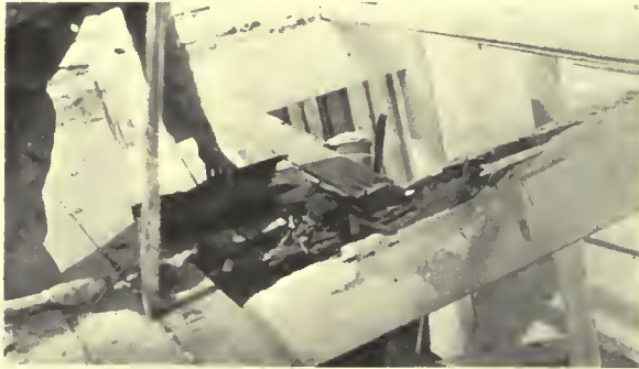
Fig. 9. Ends of roof planks rotted over the supporting beam. The rot has also extended three or four inches into the beam.
