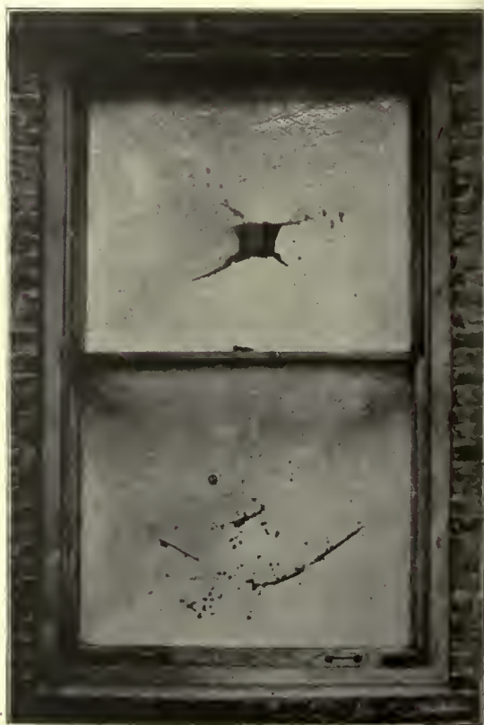
A new type of fire window without any muntins, approved for certain locations.
