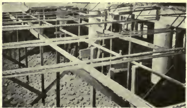
View looking down on first floor. False work for supporting forms already in place.
