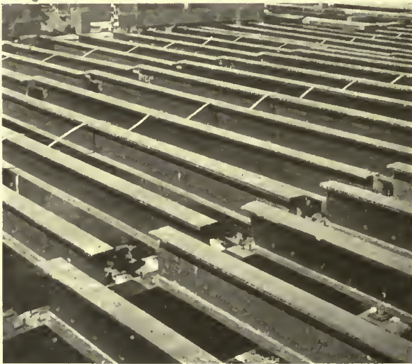
Floor construction in a large apartment house, metal joists supported on structural steel girders, galvanized iron bridging strips in place.
