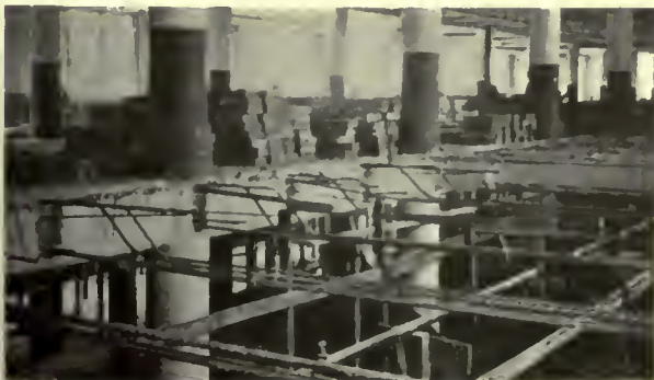
Condition of outer bay after concrete had been removed. Note beam reinforcing rods left in place; also that cases of sheet tin stacked in center panel are located over girders.
