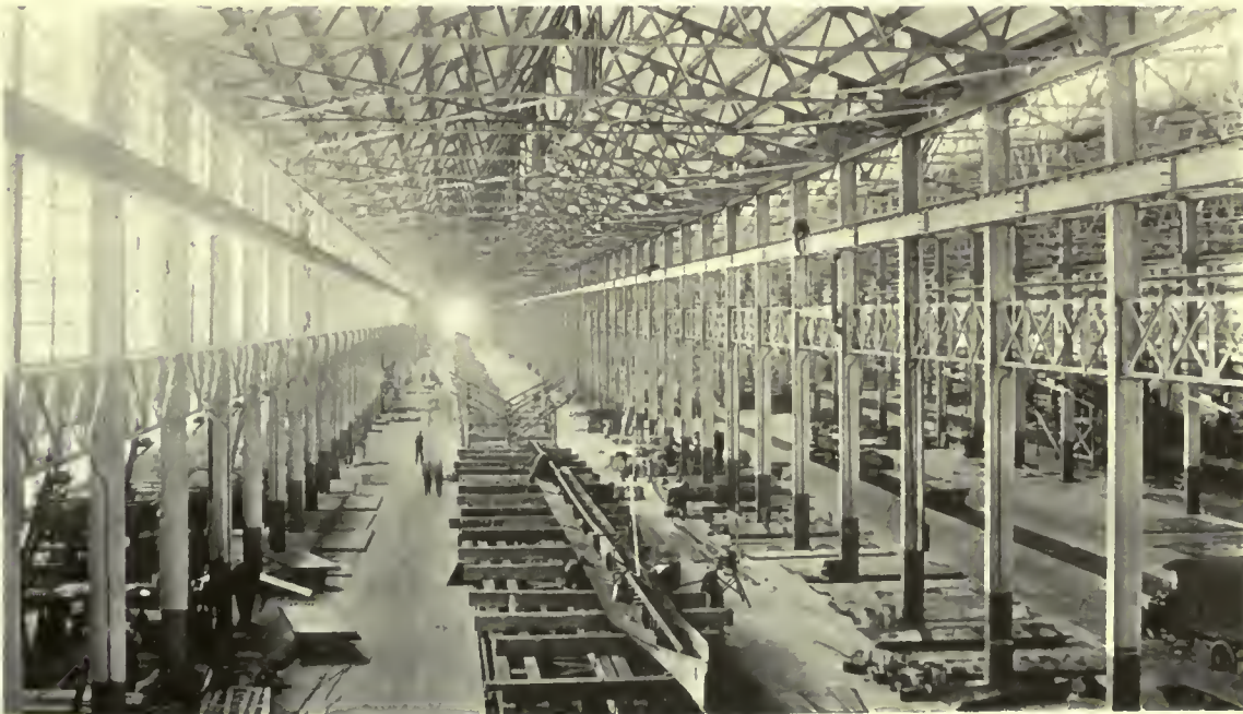
Assembling shop showing one of the five main bays and a low side bay. Note the fine daylighting.
