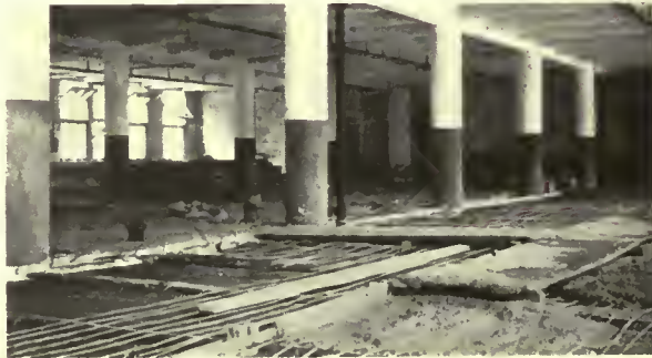
New slab being placed. Reinforcing rods showing are those taken out of demolished floor slab, straightened and re-used.
