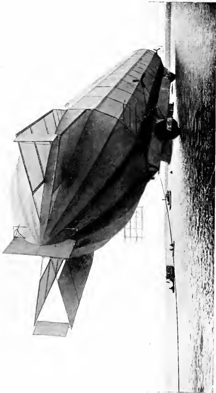
STERN VIEW OF "ZEPPELIN IV," SHOWING THE PLANES AND RUDDERS. THE PROPELLERS ON THE RIGHT SIDE CAN ALSO BE SEEN
