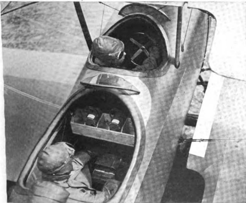
FIG. 36.—Training plane equipped for photography, showing "L" camera in floor mount and magazine rack forward of the observer.
