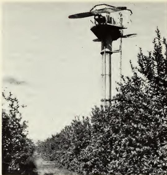
Fig. 12-1. Typical dual-engine wind machine in a citrus orchard.
