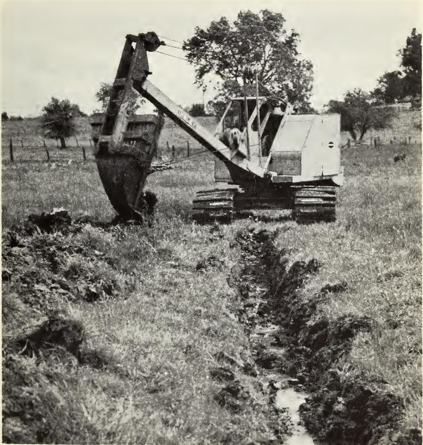
Fig. 10-9b. Back hoe digging an open drainage ditch in North Dakota.
