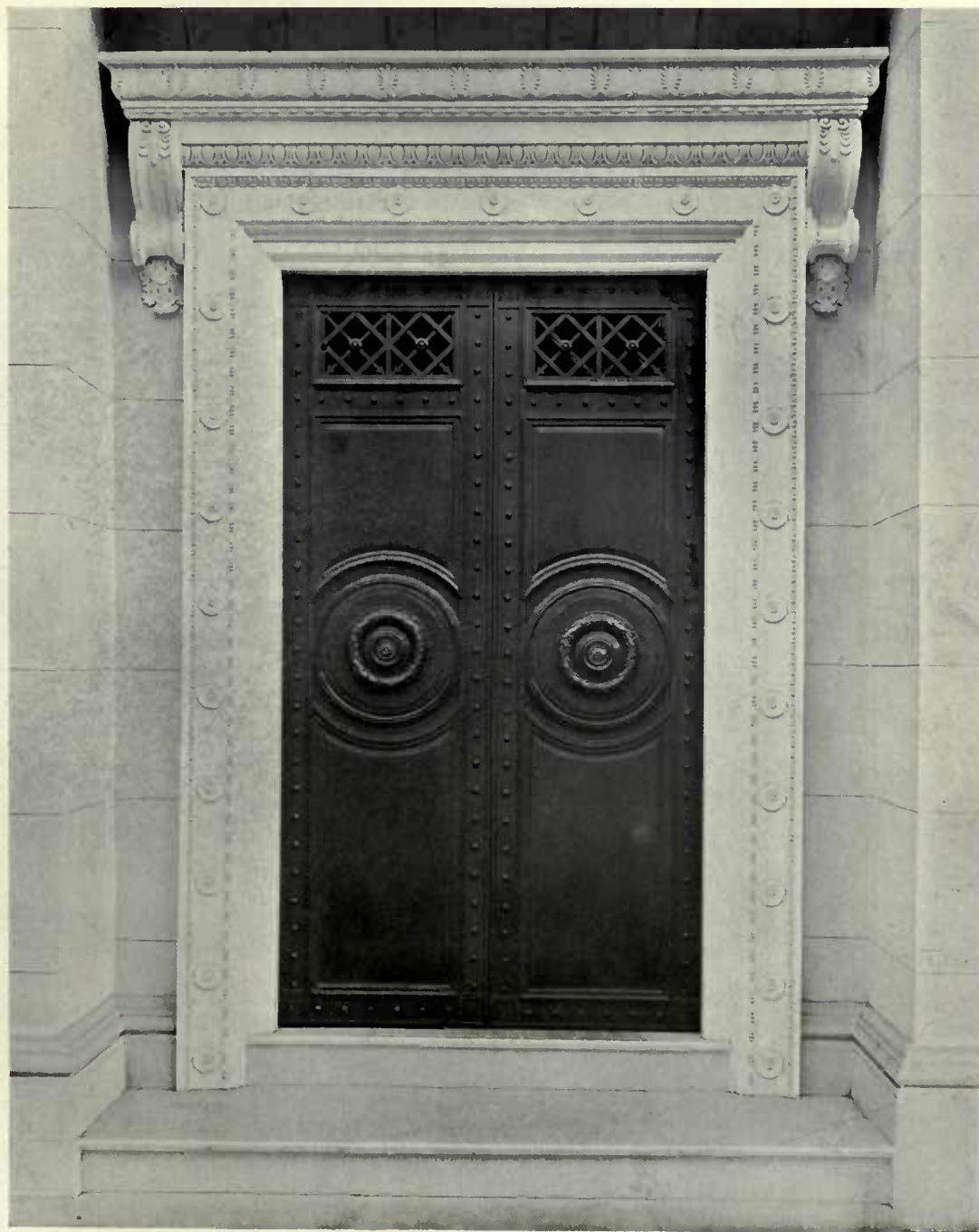
Doorway, Central Heating Pavilion.
