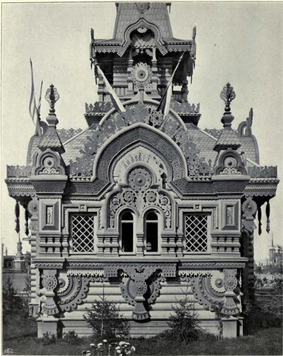
Exhibition Building, Nishny Novgorod, 1896, A. GRIGORIEFF, Architect.
