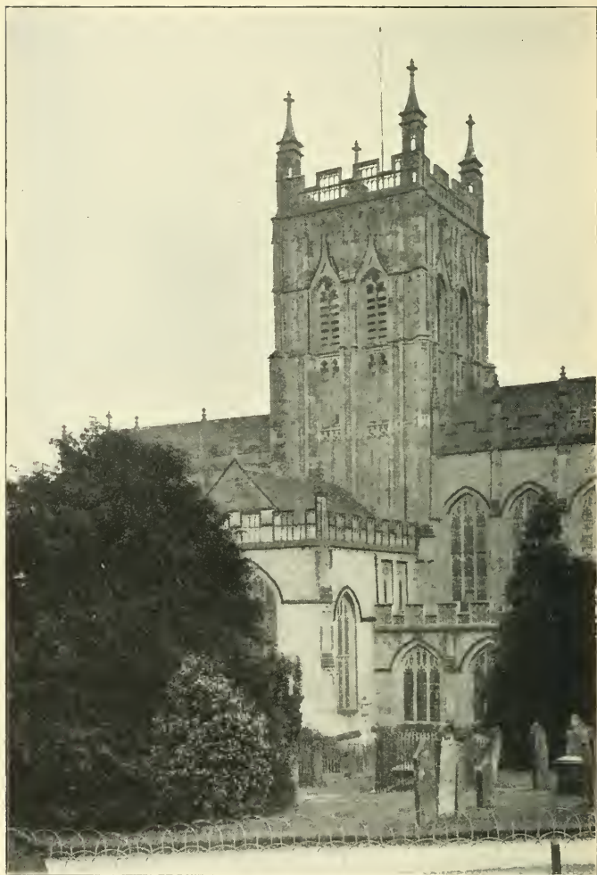
EXTERIOR, FROM NORTH-WEST
