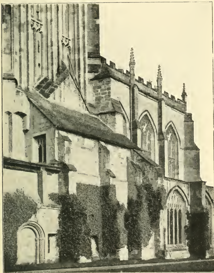
EXTERIOR, SOUTH SIDE, 1 SHOWING BLOCKED NORMAN DOOR TO CLOISTERS
