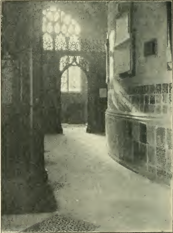
AMBULATORY AND WALL OF APSE, WITH ENTRANCE TO ST. ANNE'S CHAPEL
