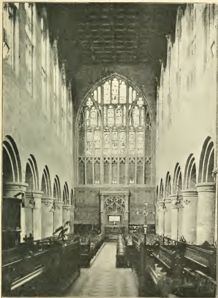
INTERIOR, WEST VIEW
