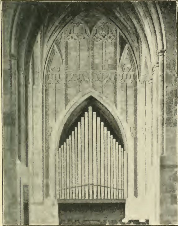
PANELLING UNDER THE SOUTH TOWER ARCH
