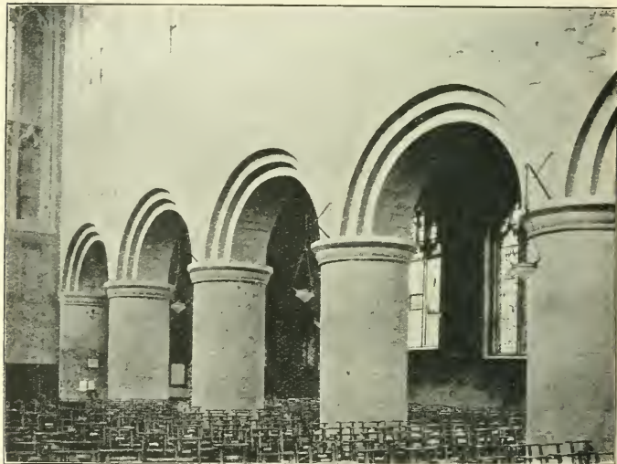
THE NAVE, LOOKING NORTH-WEST
