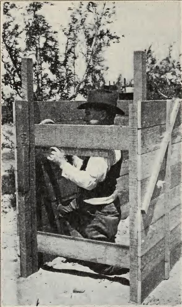
Fig. 9.—Assembling side-wall forms and placing the  $1 \times 6$  inch cross ties in the proper position.
