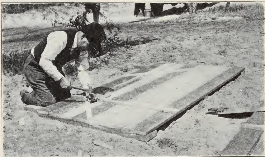
Fig. 8.—Nail the 1 × 2 inch baffle cleats firmly in position after trimming the side-wall sheathing.
