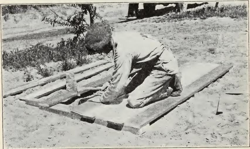
Fig. 7.—The side-wall sheathing should be well nailed, and the boards drawn close together.
