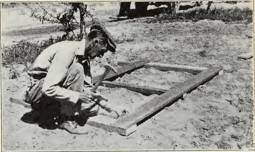
Fig. 6.—Squaring up and starting the side-wall form.
