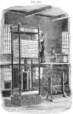
The quantity of liquid which is necessary to force the plunger and platform up, is small, and the pressure exercised by it very strong (from 200 to 500 tons); the pumps may therefore work slowly, and their channels may be very small, but their bodies must be able to withstand a heavy pressure.
