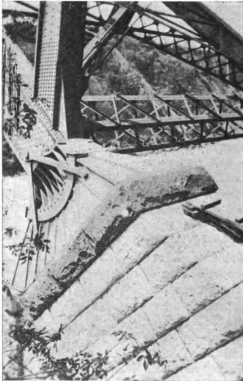
FIG. 246.—NIAGARA SKEWBACKS AS BUILT.
