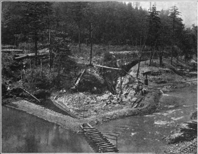
FIG. 21.—GREEN RIVER LOG CRIB COFFER-DAM.
