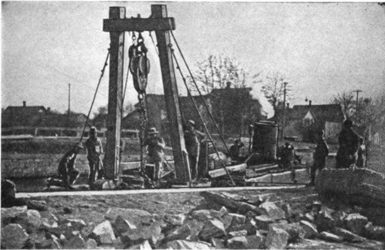
FIG. 51.—PILE-PULLING SCOW, NEW YORK STATE CANALS.
