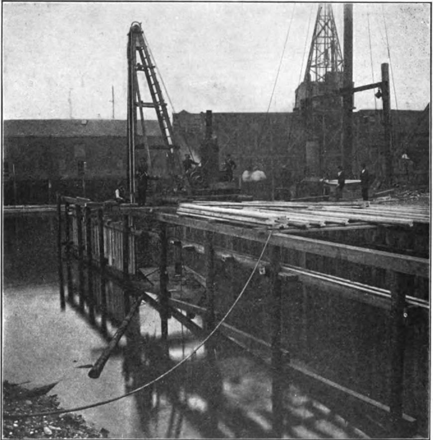
FIG. 53.—CHARLESTOWN BRIDGE. DRIVING WAKEFIELD SHEET-PILING.
