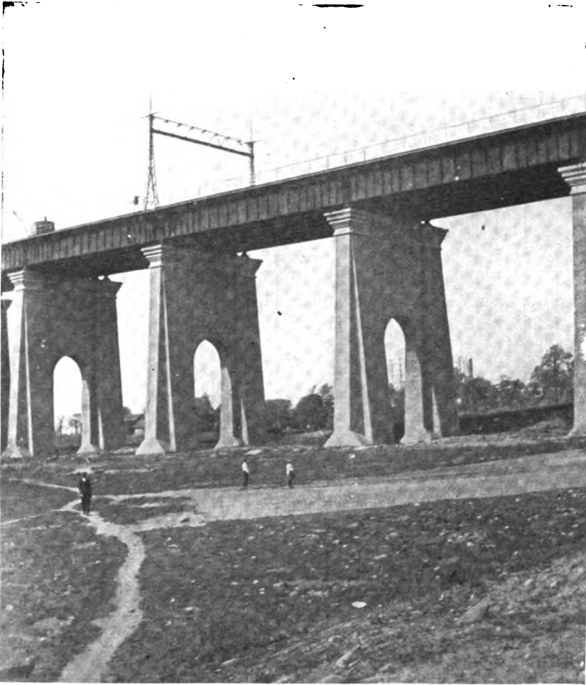
FIG. 264.—HELLGATE APPROACH PIER.
