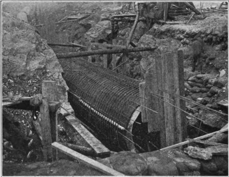
FIG. 22.—PLACING REINFORCED PIPE, GREEN RIVER COFFER-DAM.
