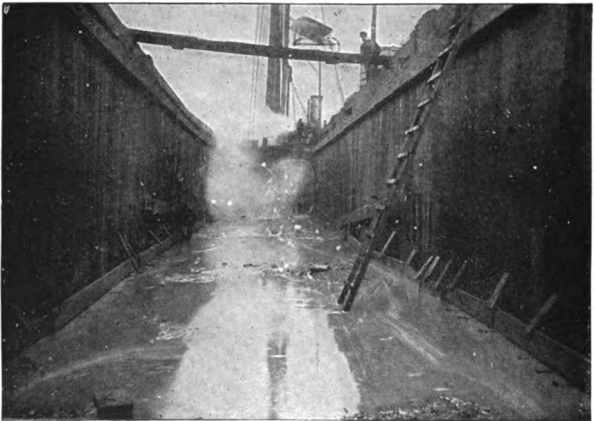
FIG. 86.—COFFER-DAM ON CHARLESTOWN BRIDGE.
