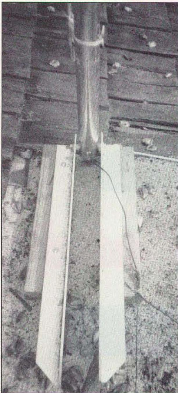
Photo D. The Voyager's hinged base allows for an "easy" tilt-up.
