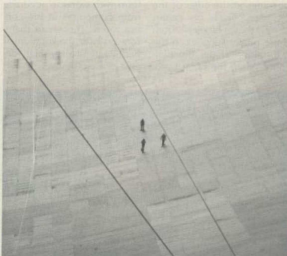
Workmen on the reflecting dish are using shoes which distribute their weight over a large area, like snowshoes. Walking on the reflecting dish is now being avoided, and almost all adjustments and repairs are being done from the underside.
