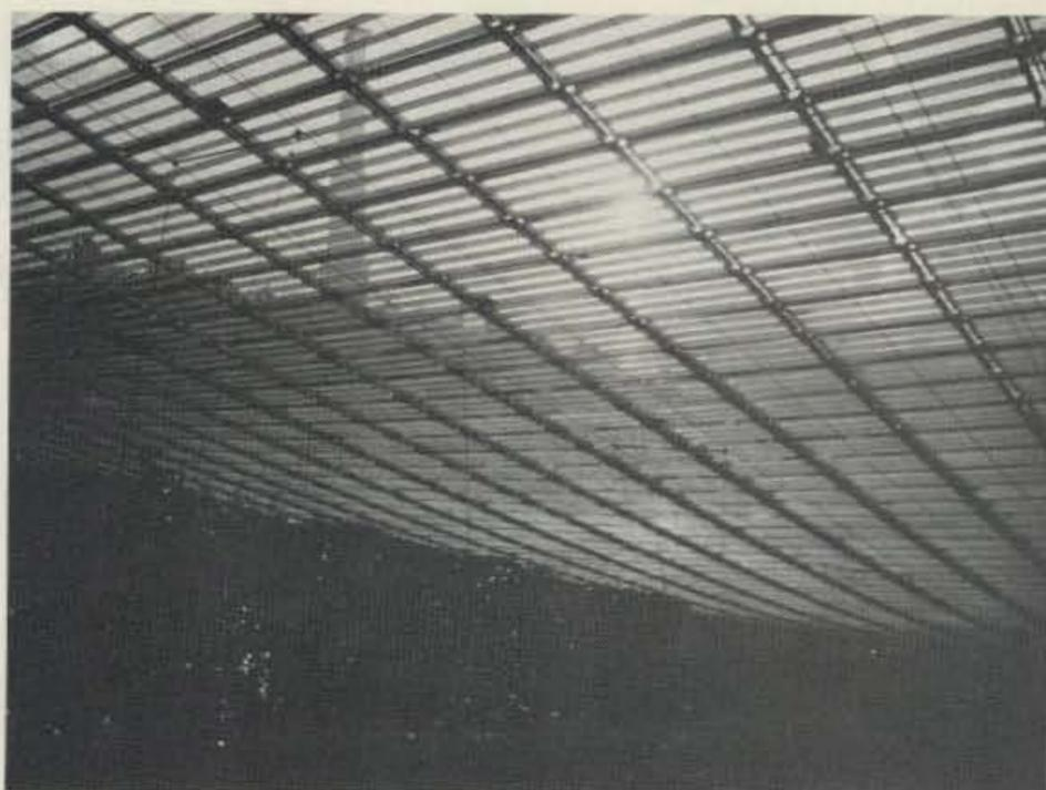
The aluminum panels are perforated so that much of the sunlight can pass through. Vegetation can therefore grow under the reflecting dish, preventing erosion of the landscape.
