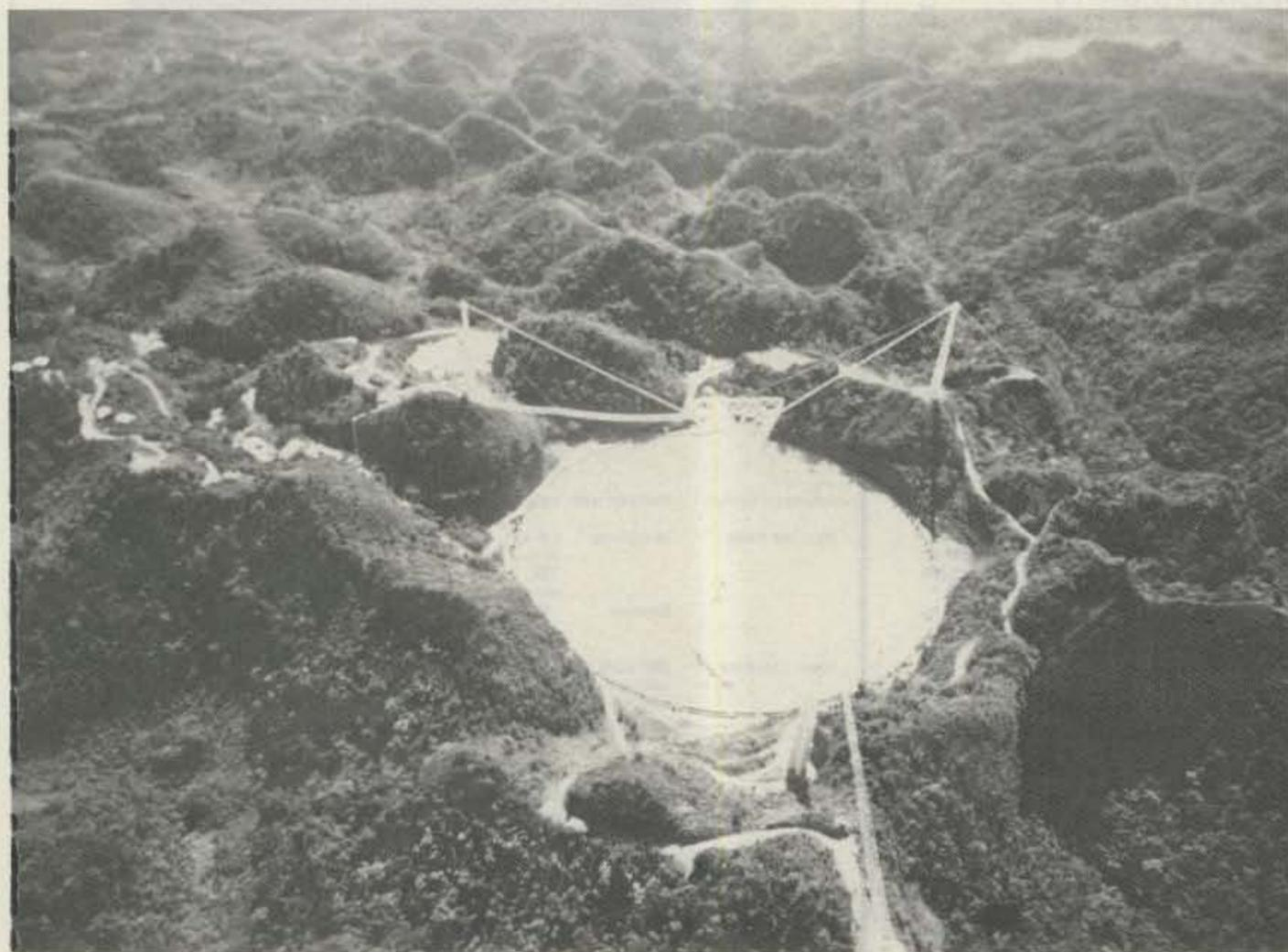
*The 1000-foot reflecting dish at Arecibo was built in a natural limestone sinkhole.*
