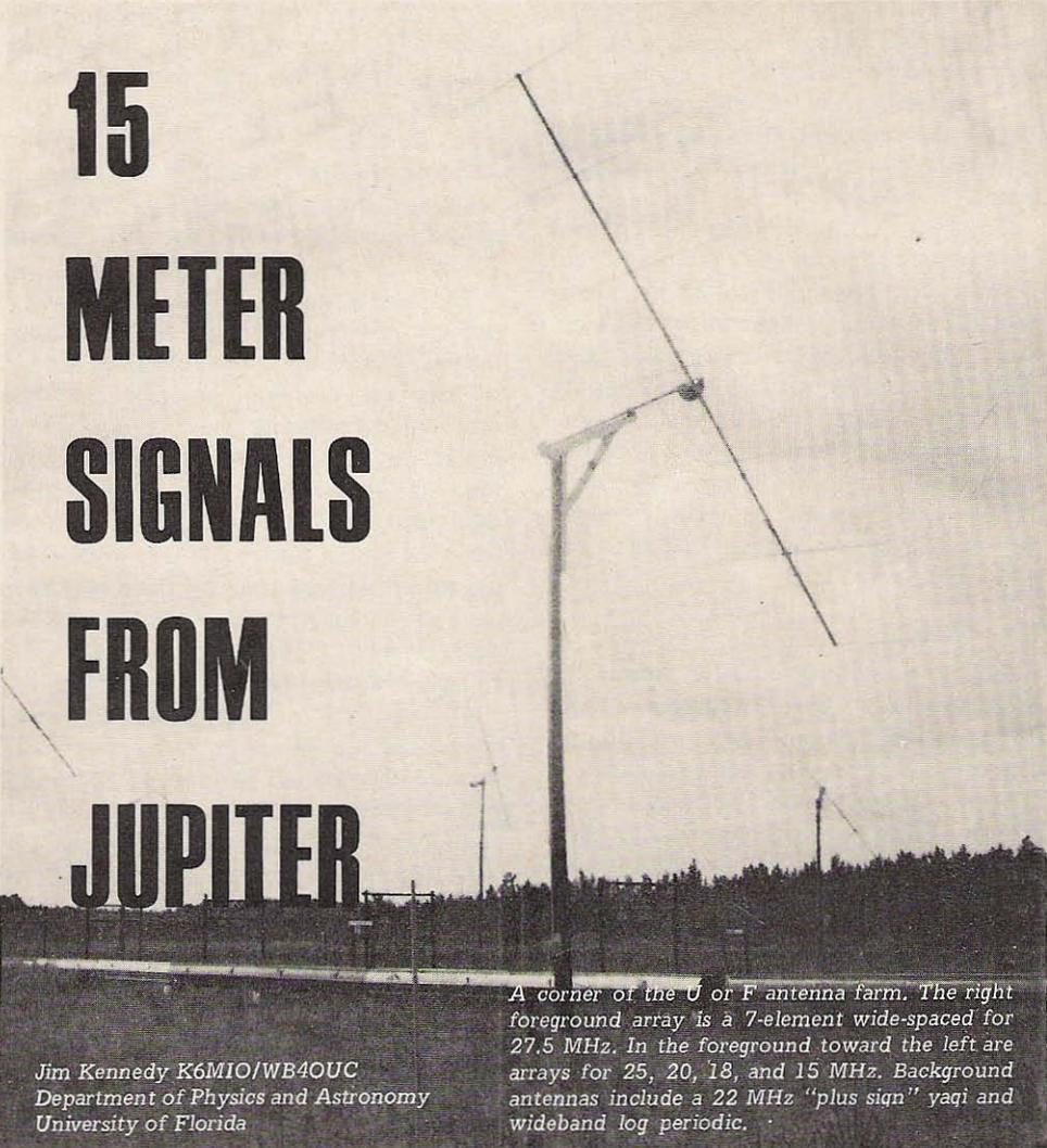
A corner of the U or F antenna farm. The right foreground array is a 7-element wide-spaced for 27.5 MHz. In the foreground toward the left are arrays for 25, 20, 18, and 15 MHz. Background antennas include a 22 MHz "plus sign" yagi and wideband log periodic.
