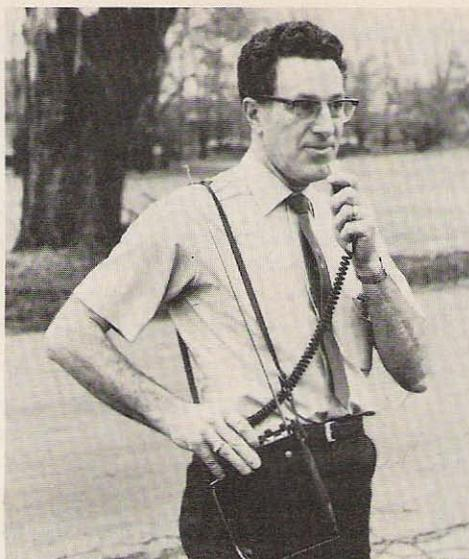
As a portable unit, the TR-22 operates from its own self-contained batteries. A carrying case and shoulder strap are provided with the unit, as is the pencil microphone with its curl cord. Power output is between 1.1 and 1.5W, depending on condition of batteries.
