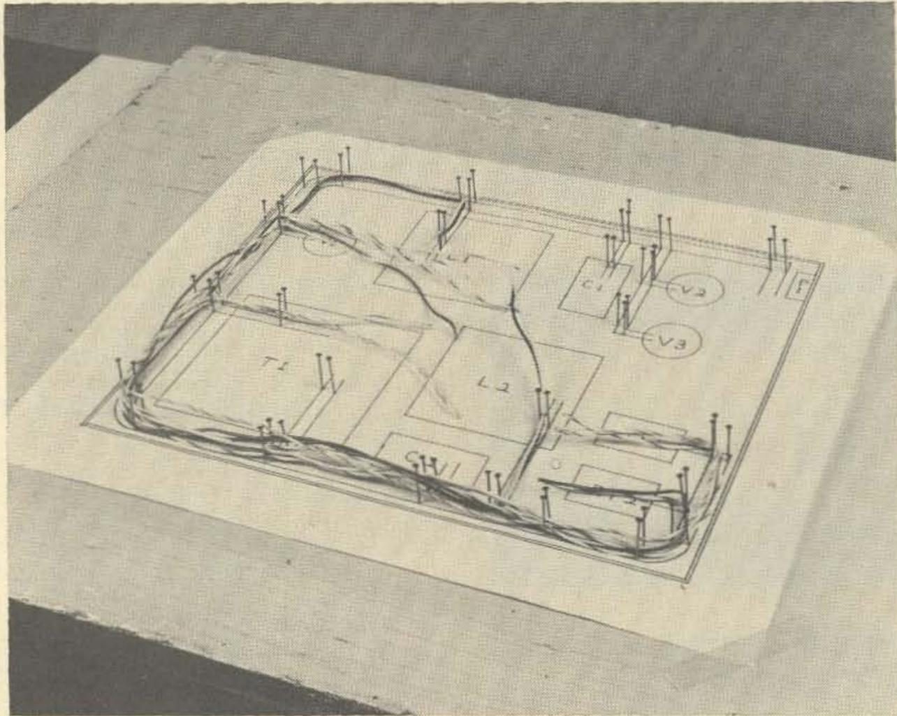
When building any complex piece of electronic equipment, you will usually find that the majority of the wiring consists of power and control wiring of one kind or another. This wiring is usually completely uncritical as to length and placement, so ordinarily not much thought is given to its installation. Any method of wiring may work well electrically, but later on, when it is necessary to trouble-shoot the circuit and make repairs, you may find that you have built-in some unnecessary troubles.
