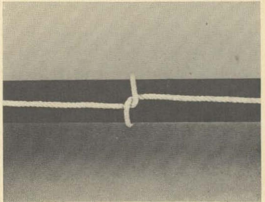
*The proper method of lacing.*
