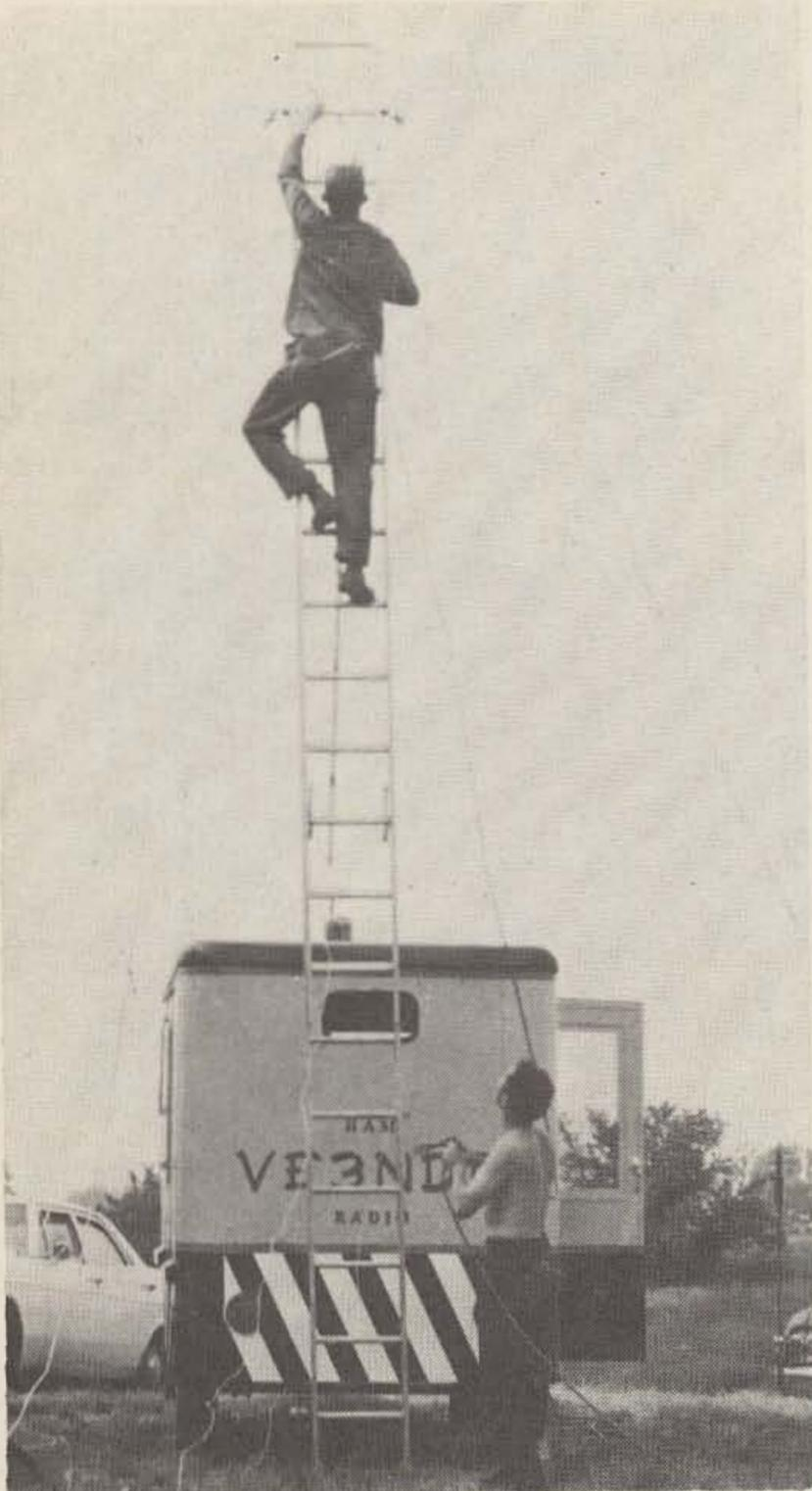
VE3DNR on a field day site. A 40-foot aluminum ladder is used as an antenna mast.
