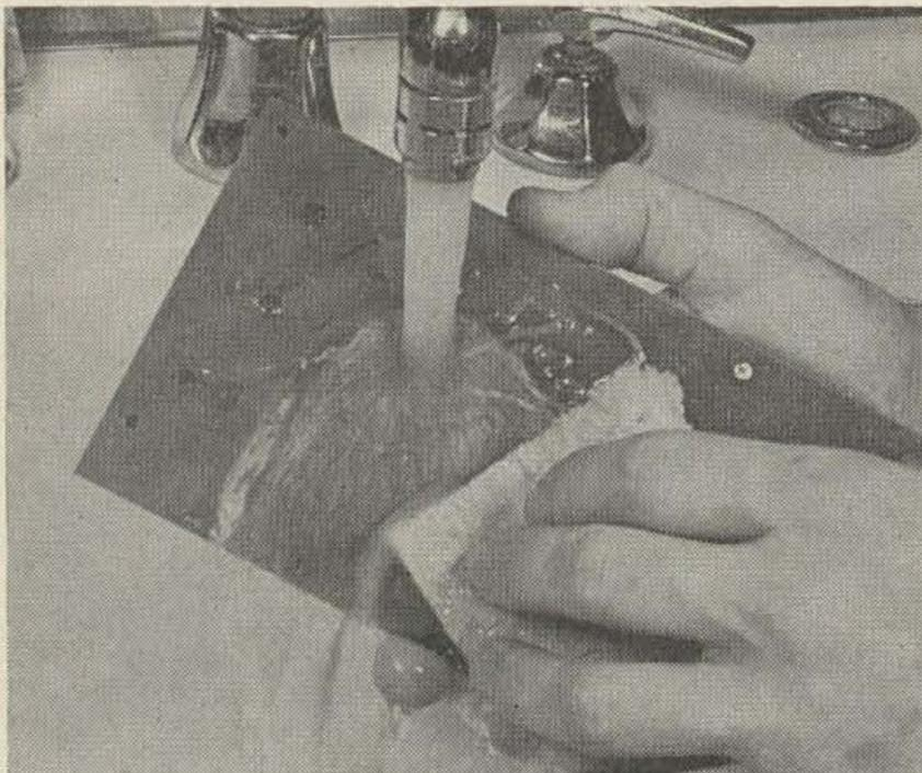
10—Board is removed immediately when all excess copper has been removed, and is thoroughly rinsed to eliminate all traces of etchant.
