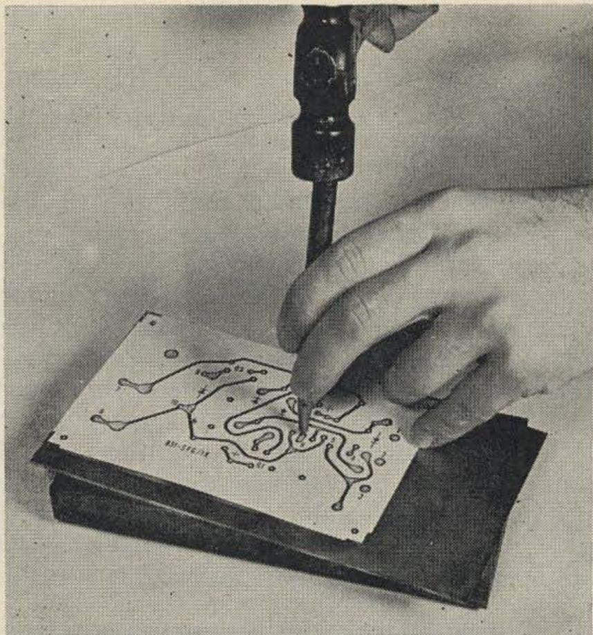
4—Allow to dry, then lightly punch the centers for holes to be drilled later.
