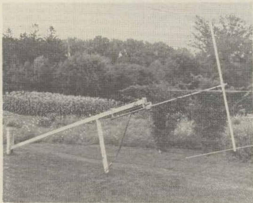
Fig. 2. Mast pivots over for work. 2" x 4" used as a prop.
