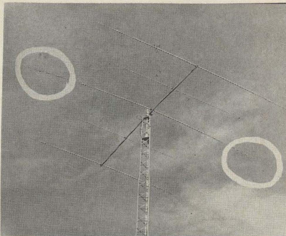
VIEWS OF TRI-BAND ANTENNA AT WOJRQ IN DENVER, COLORADO, WITH "SPACE-GUNS" ADDED FOR 40 METERS
