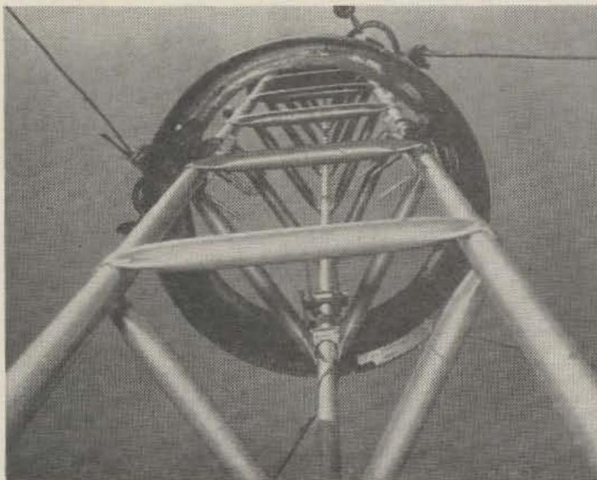
does not seem to be harmful. The horizontal force bears on the bolt heads which hold the roller skate wheels in their carriers. The rubbing of these bolts against the inside of the ring might make necessary their replacement every few years. Even so the tower runs quite freely with very little binding as long as the guys are kept somewhat loose. They tend to grow taut in cold weather.
