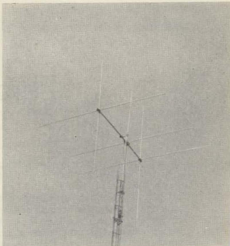
Hailed by HF men as a major break through in antenna design and performance, the famous K6CT polarized diversity beam, based on the proven principles of the Yagi parasitic array and Brown turnstile antennas, and using the rugged plumbers delight construction.
