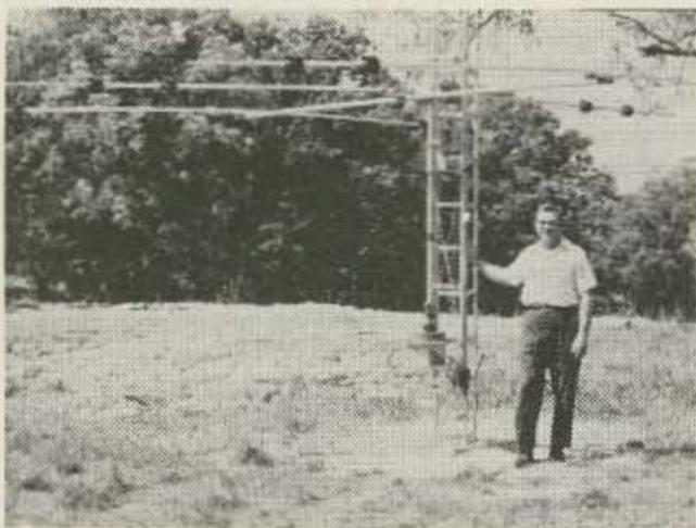
We hope you can see in the photo how the array and the rotator both go up and down the Hy-Track on rails. When you crank it to the top it locks in place. It automatically unlocks when you want to lower it again. Note how little ground area is needed.
