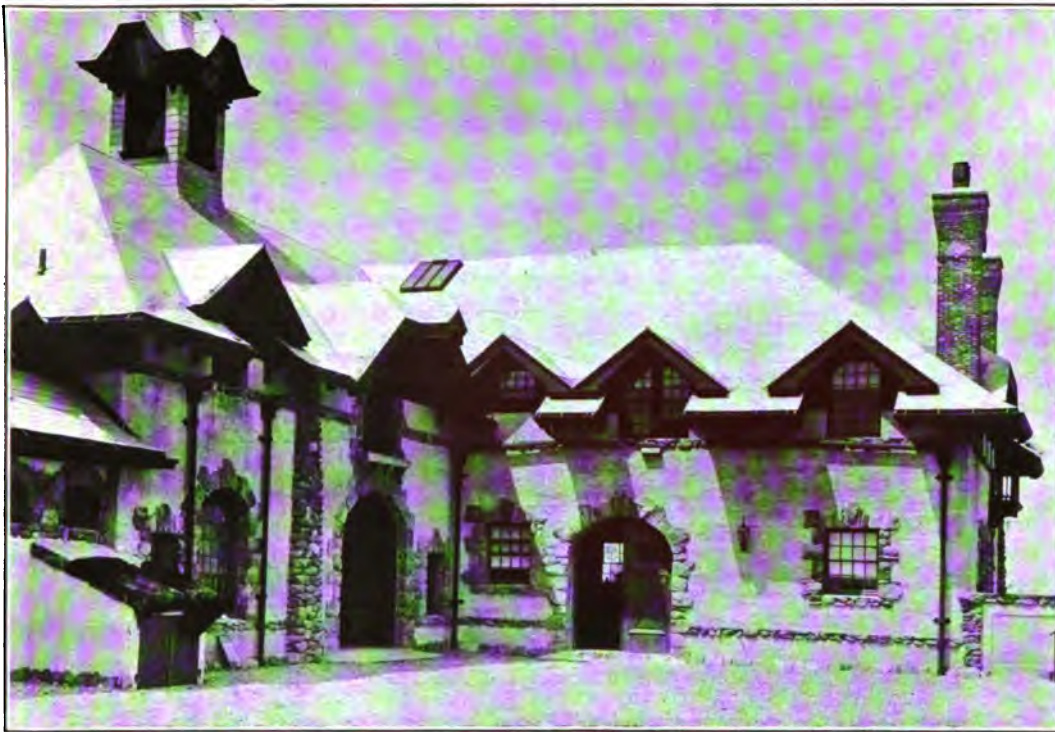
REINFORCED CONCRETE STABLE, WITH ASBESTOS "CENTURY" SHINGLE ROOF, BUILT BY SIMPSON BROS. CORPORATION FOR THEODORE M. DAVIS, NEWPORT, R. I.
