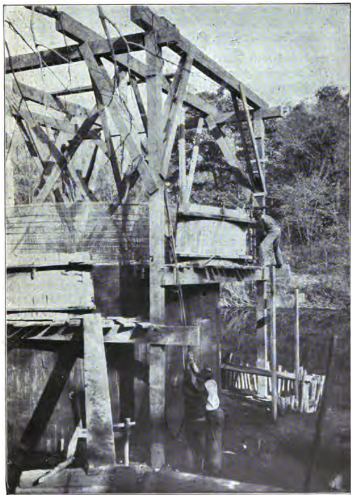
Fig. 155.—Manner of Raising Forms, Intake Tank, LaSalle, Ill.
