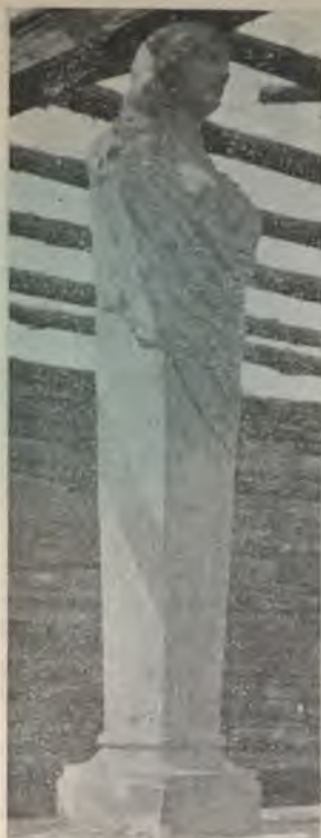
FIG. 97.—ONE OF A NUMBER OF SYMBOLIC FIGURES IN CONCRETE, FORMING SUPPORTS FOR RESTIC PERGOLA, ESTATE OF ALBA B. JOHNSON, ROSEMONT, PA.—ADOLPH SCHILLING
