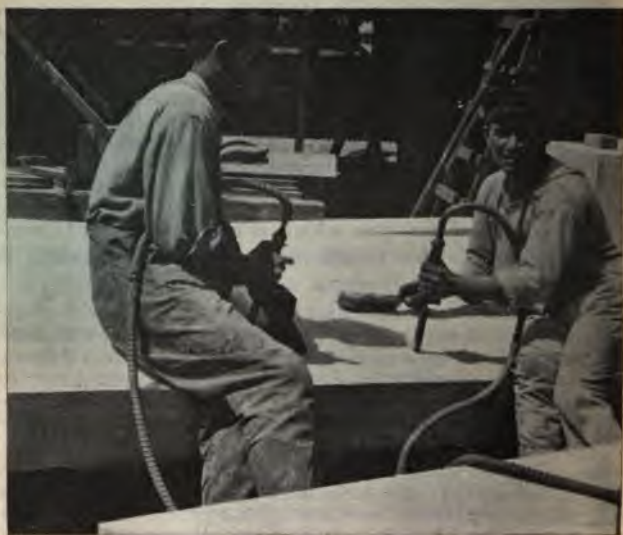
FIG. 79—USING PNEUMATIC TOOL IN FINISHING CONCRETE.
