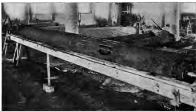
FIG. 50—MAKING HOLLOW REINFORCED CONCRETE COLUMN BY MEANS OF MANDREL
