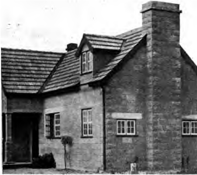
FIG. 94—DETAIL, CONCRETE BLOCK COTTAGE, WAYFORD WOOD ESTATE, NORFOLK, ENGLAND
