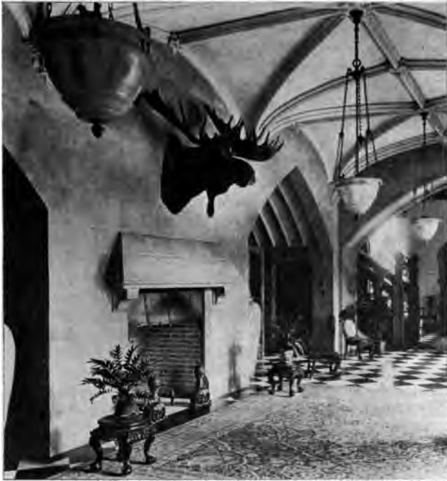
FIG. 7.—INTERIOR OF RESIDENCE CONCRETE STONE, NEW HAVEN, CONN.—NEW ENGLAND STONE CO.
