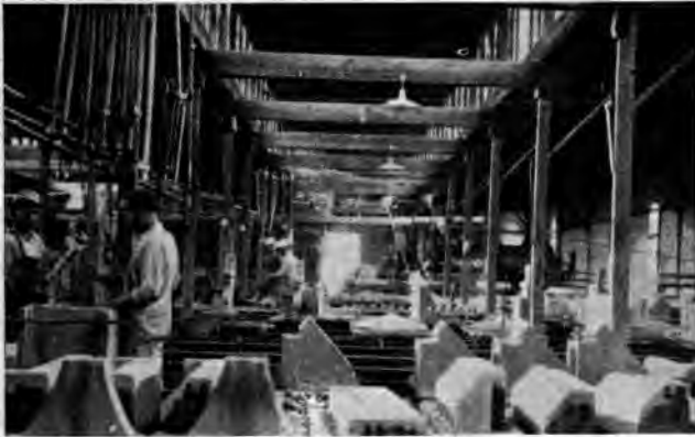
FIG. 37—VIEW OF MOLDING ROOM OF TRIM STONE FACTORY—NOTE MOLD BEING FILLED AND CONCRETE TAMPED AT LEFT
