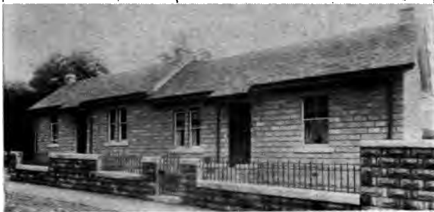
FIG. 5.—TWO-FAMILY CONCRETE BLOCK COTTAGE AT DUNBARTON, SCOTLAND.
