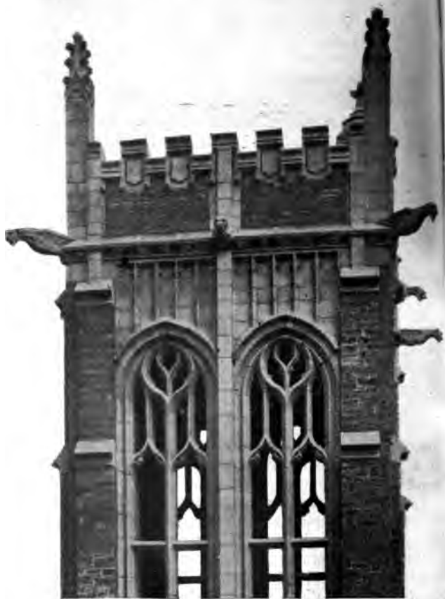
FIG. 93—CONCRETE STONE TRIM, TOWER, BROADWAY PRESBYTERIAN CHURCH NEW YORK CITY—ONONDAGA LITHOLITE CO.
