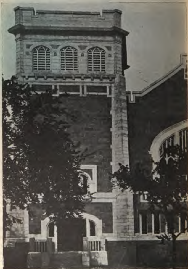
FIG. 95—CONCRETE BLOCK (GRAY CEMENT) AND CONCRETE STONE TRIM (WHITE CEMENT), NORMAL PARK, M. E. CHURCH, CHICAGO
