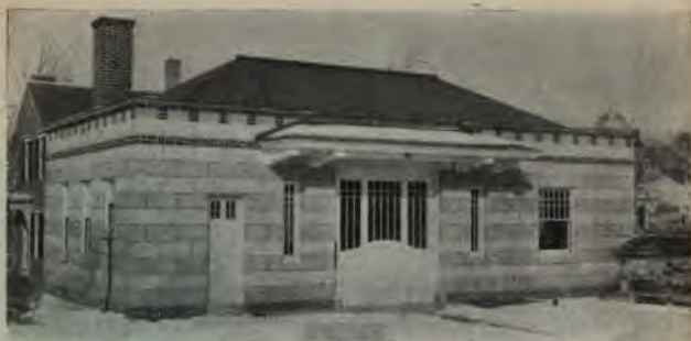
FIG. 6—CONCRETE VENEER BLOCK IN GARAGE, NEW BEDFORD, MASS.—STURTEVANT & HOOK.
