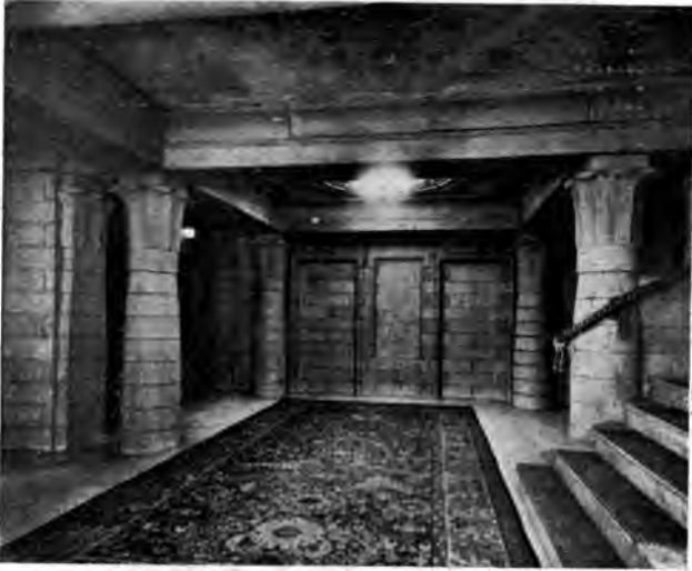
FIG. 4—ELEVATOR FOYER, BASEMENT, HOLLENDEN HOTEL, CLEVELAND— GEORGE RACKLE & SONS CO.
