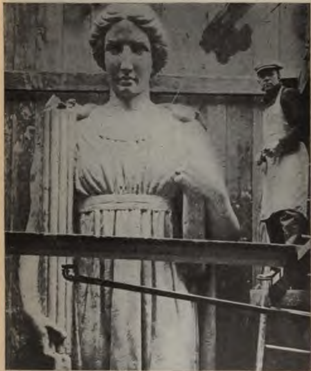
FIG. 43—FINISHING CLAY MODEL 16' HIGH FOR CONCRETE STATUE
