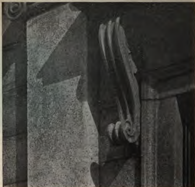
FIG. 74—SMALL DETAIL OF GRANITE CONCRETE MAUSOLEUM, RUBBED FINISH —CHARLES EILBACHER
