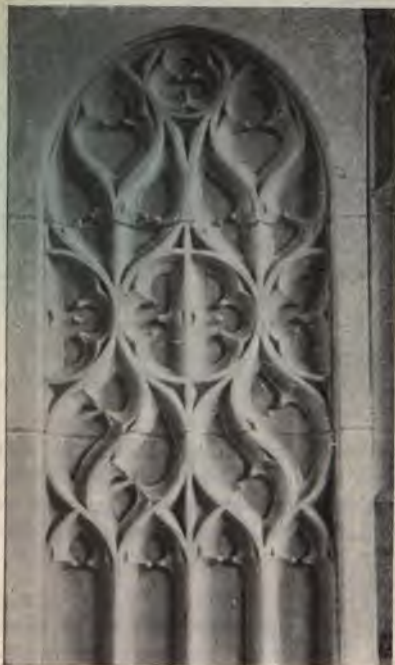
FIG. 40—SMALL CONCRETE PANEL, PART OF CHURCH ALTAR, MADE IN PLASTER MOLD
