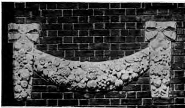
FIG. 81.—DETAIL OVER ENTRANCE—SAND-CAST CONCRETE, CARVED AFTER SETTING—ONONDAGA LITHOLITE CO.
