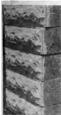
FIG. 65—COMMON VARIETY OF WHITE ROCK-FACE BLOCK
