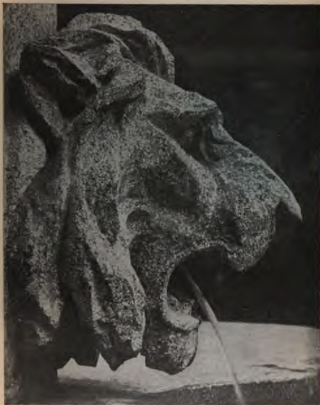
FIG. 75—SAND-CAST CONCRETE, HAND-TOOLED—EMERSON & NORRIS CO.
