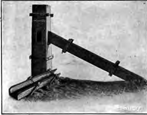
Fig. 559.—View of Mould for Corner Post.
