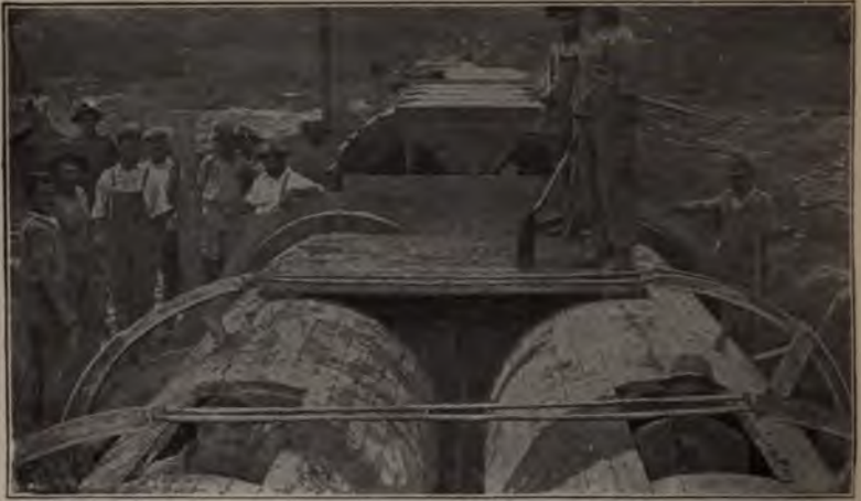
Fig. 482.—Forms for Double Conduit, Cedar Grove Reservoir.
