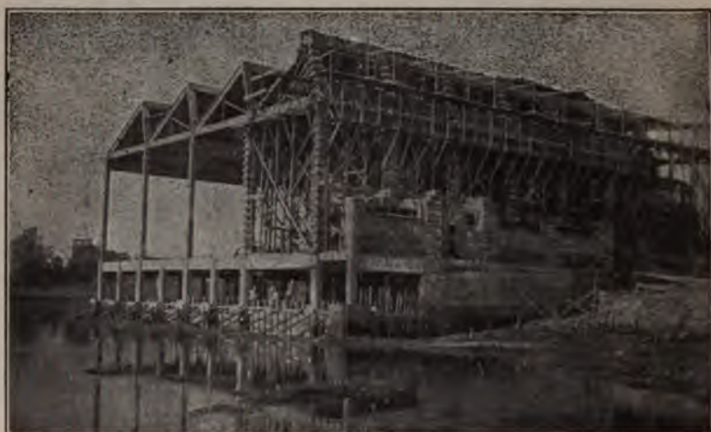
Fig. 378.—View of Factory at Stamford, Conn., Under Construction.
