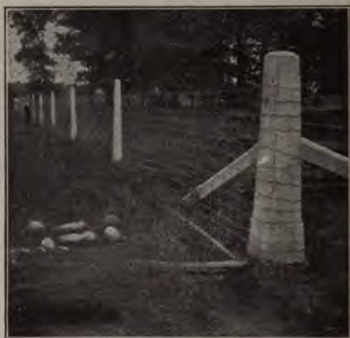
Fig. 558.—View Showing Reinforced Concrete Posts in Fence.
