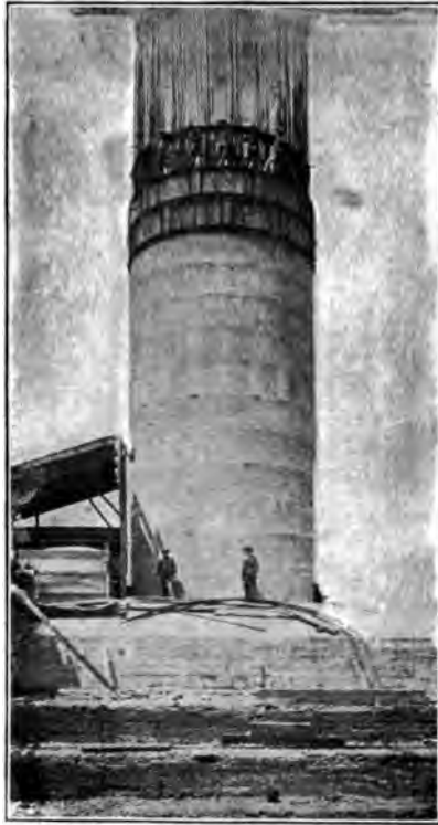
Fig. 543.—View Showing Forms for Weber Chimney.
