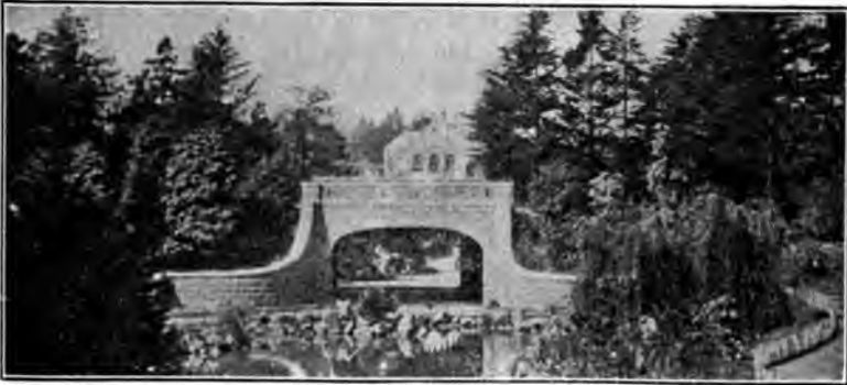
Fig. 2.—Reinforced Concrete Arch Bridge built in 1889, at Golden Gate Park, San Francisco, Cal.
