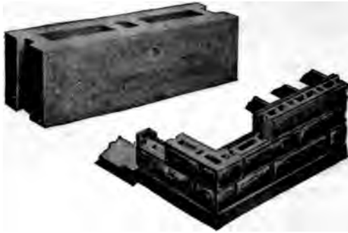
Fig. 698.—Examples of Harmon S. Palmer's Hollow Concrete Blocks.
