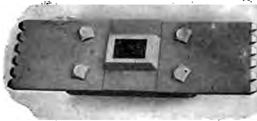
Fig. 57.—Ransome Ax for Dressing Concrete Surfaces.
