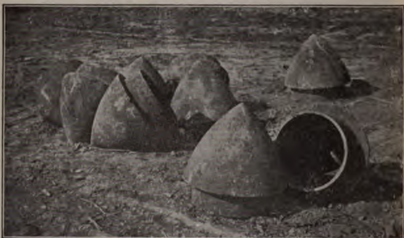
Fig. 243.—Cast Iron Points for Simplex Piles.
