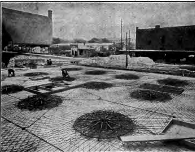
Fig. 315.—View of Floor, Mushroom System of Construction.
