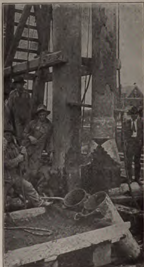
Fig. 245.—Simplex Pile Driver and Alligator Point Driving Form.
