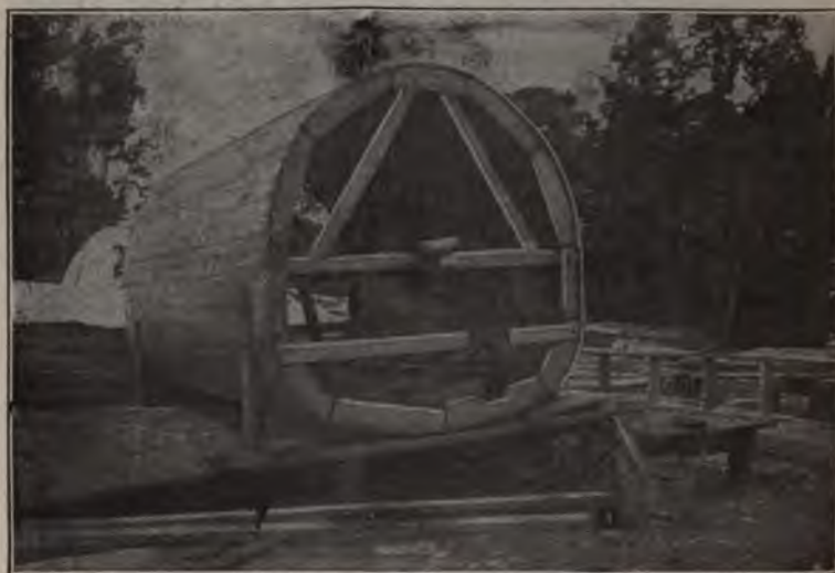
Fig. 185.—Center for Jersey City Water Works Conduit.
