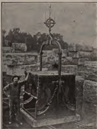
Fig. 52.—O'Rourke Concrete Bucket, Closed.
