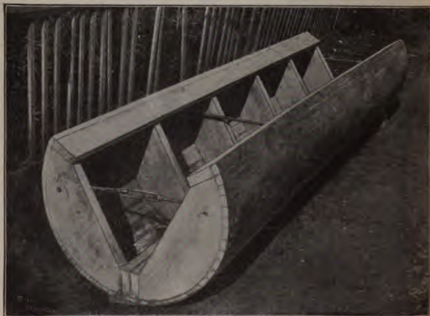
Fig. 506.—Form for Sewer Invert at Medford, Mass.
