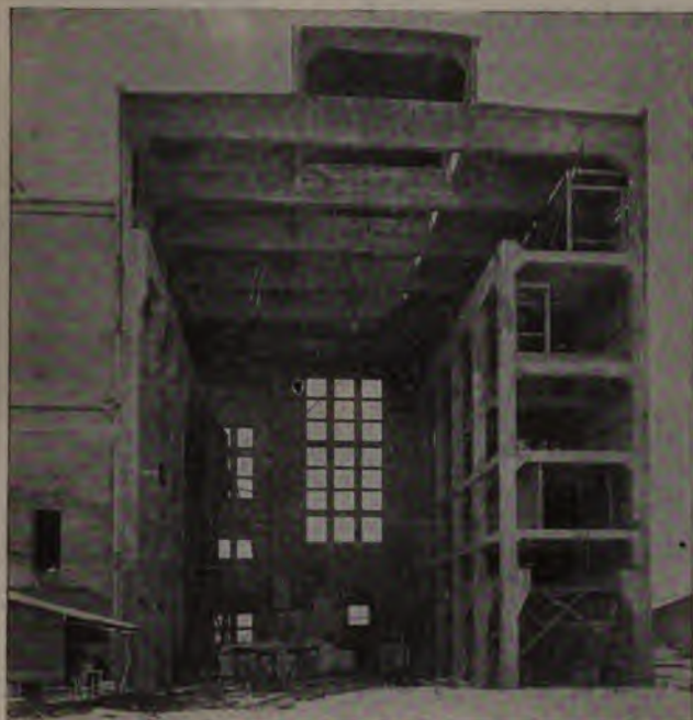
INTERIOR OF ENGINE ROOM, SHOWING 64 FOOT ROOF GIRDERS
