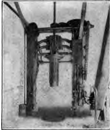
Fig. 474.—Machine Ready for Another Pipe.
