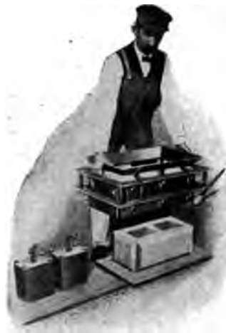
Fig. 712.—Moving the Mould Instead of the Block.
