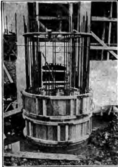
Fig. 542.—View Showing Forms for Weber Chimney.
