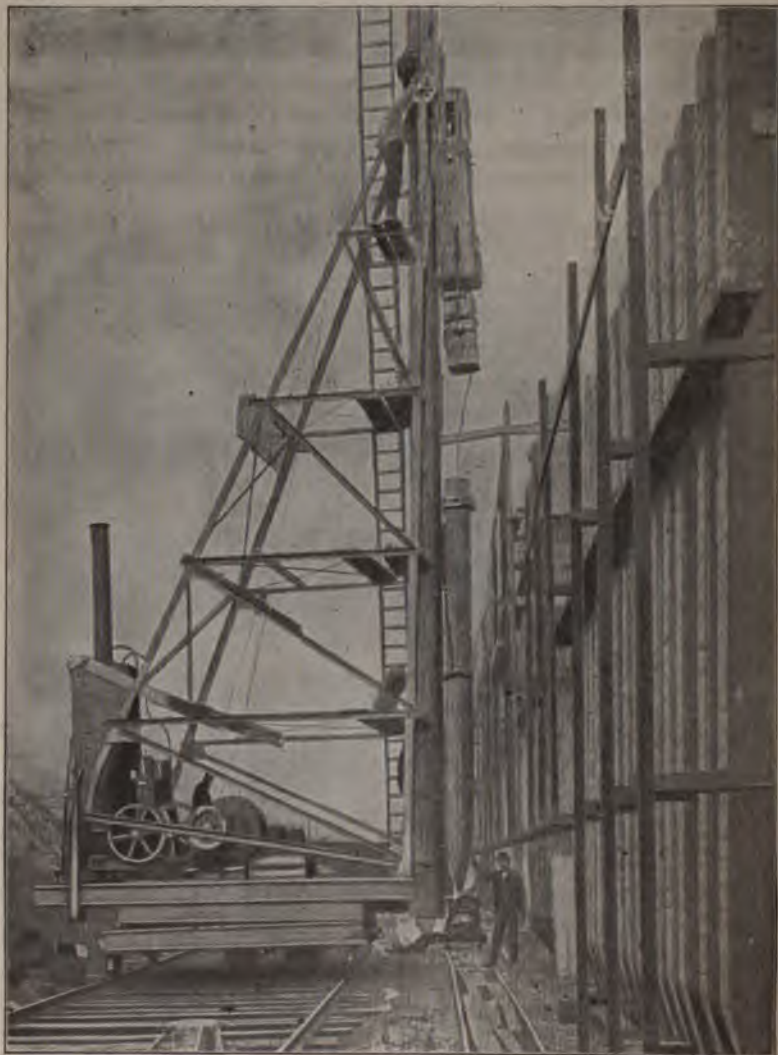
Fig. 263.—Pile Driver and Pile for Union Station, Hamburg, Germany.
