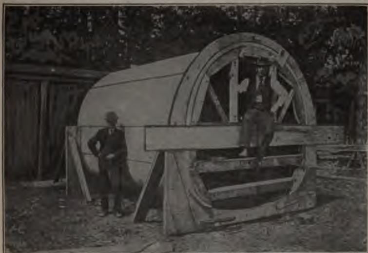
Fig. 484.—Center for Jersey City Water Works Conduit.
