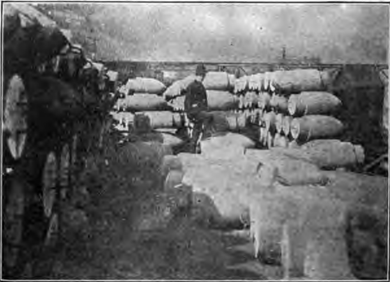
Fig. 242.—Concrete Points for Simplex Piles.
