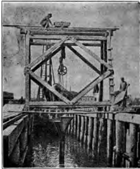
Fig. 55.—Mounting for Tremie, Charlestown Bridge Work.
