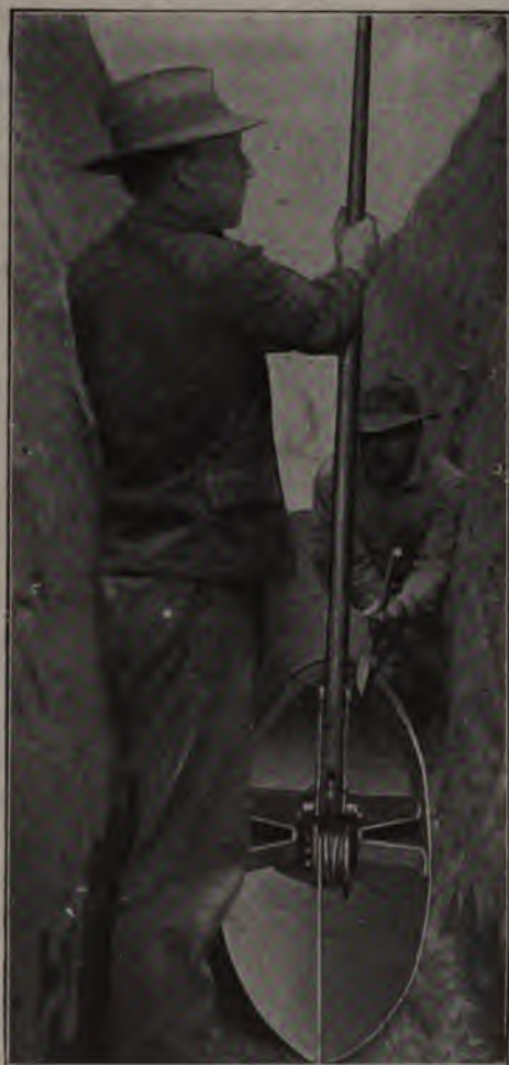
Fig. 510.—The Ransome Concrete Pipe Mold.
