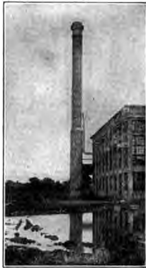
Fig. 540.—View of United Shoe Machinery Co.'s Chimney.
