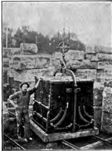
Fig. 53.—O'Rourke Concrete Bucket, Open.
