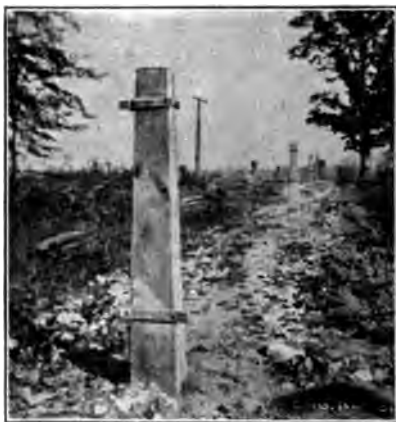
Fig. 561.—Mould for Line Post.
