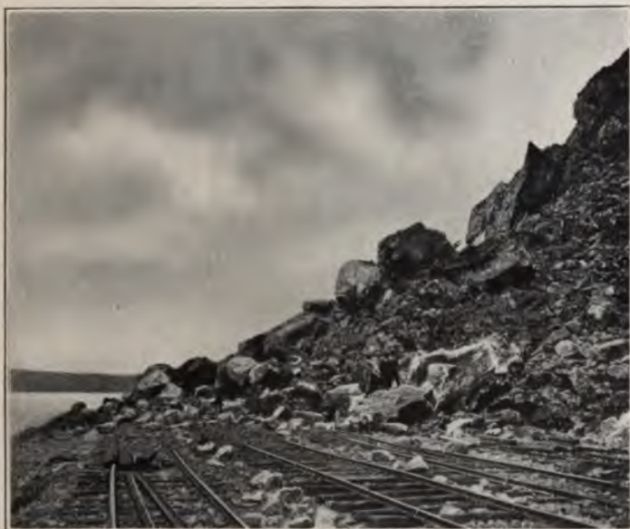
FIG. 84.—Quarrying for Fishguard Harbour. The cliffs after blasting.
