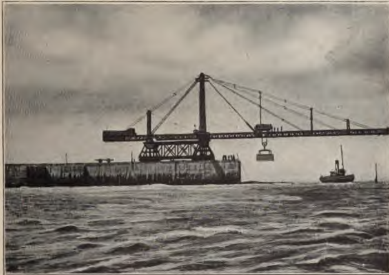
FIG. 152.—Titan at Zeebrugge Breakwater. [To face p. 178.]
